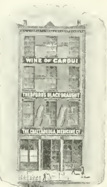
St. Louis Office and Warehouse.
