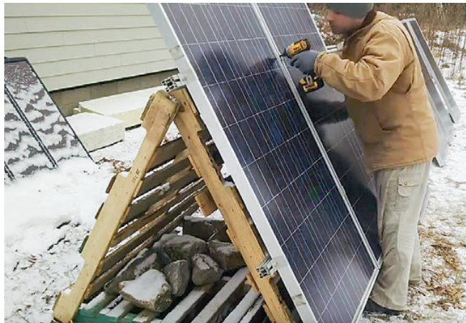
Figure 5.24 Screen capture of DIY video for solar panel mounting on pallets by David Poz.
