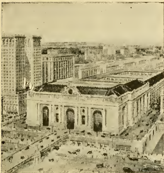
Grand Central Terminal—42nd St. and 5th Ave.
