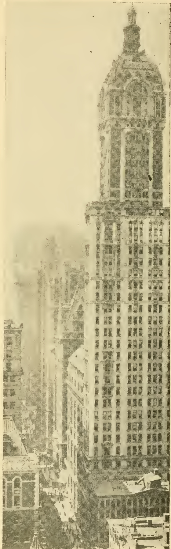
Singer Building Tower and Lower Broadway
