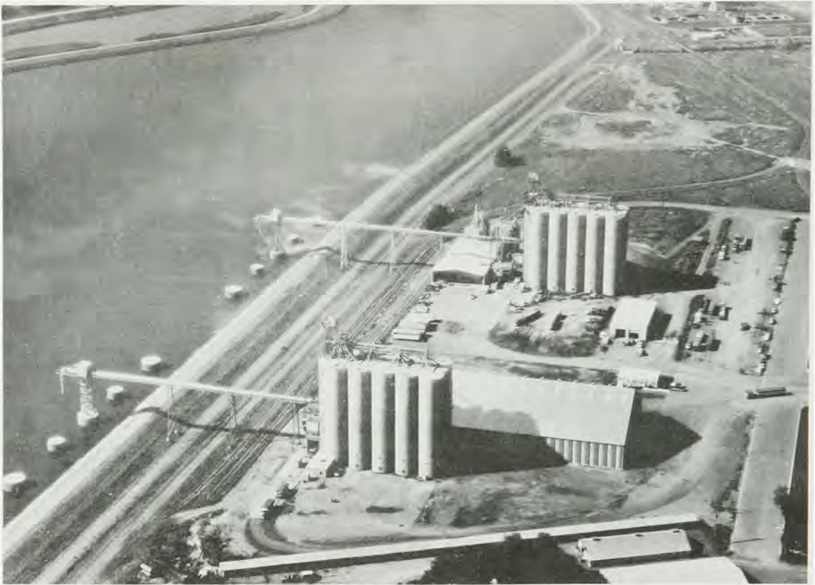
LEWISTON PORT FACILITIES
