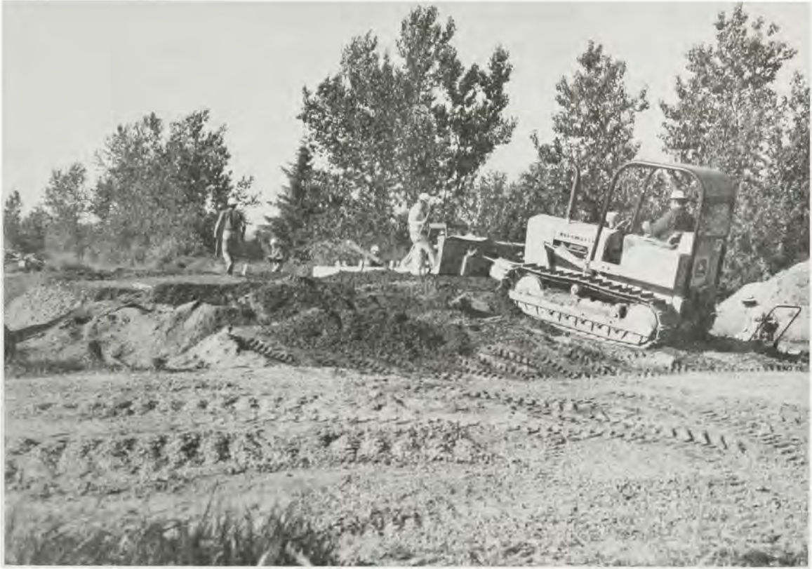
WILLOW CREEK DAM CONSTRUCTION JUNE 1980
