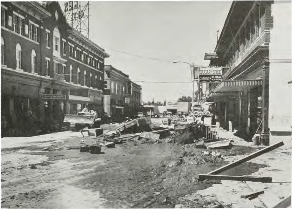
DEBRIS CLEANUP AT REXBURG
