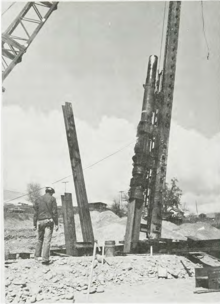
LEWISTON-CLARKSTON INTERSTATE BRIDGE UNDER CONSTRUCTION 1980
