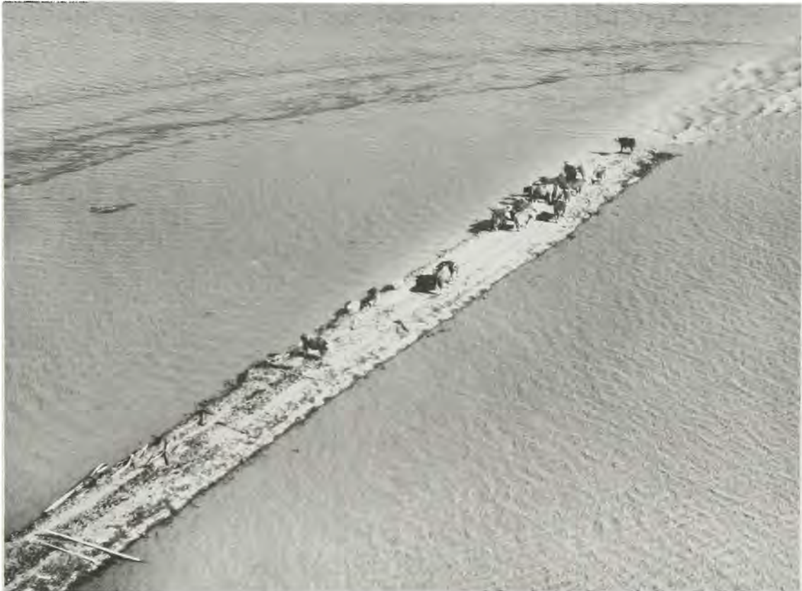
CATTLE STRANDED ON LEVEE AFTER DAM COLLAPSE
