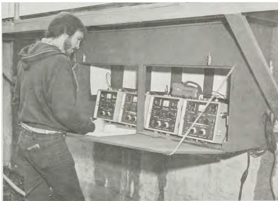
RACEWAY FISH COUNTERS AT LOWER GRANITE DAM
