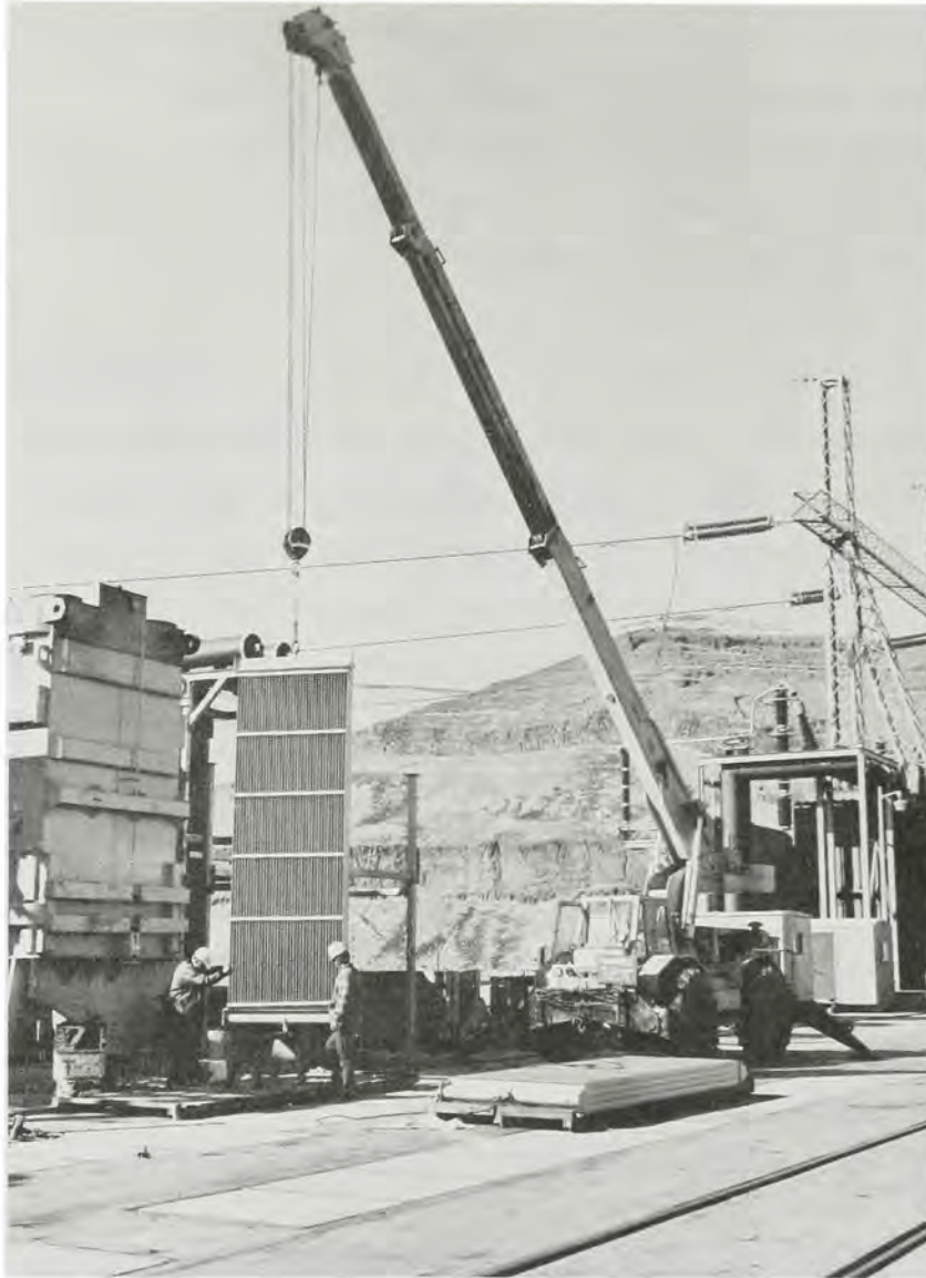
INSTALLATION OF NEW TRANSFORMER AT LOWER MONUMENTAL DAM
