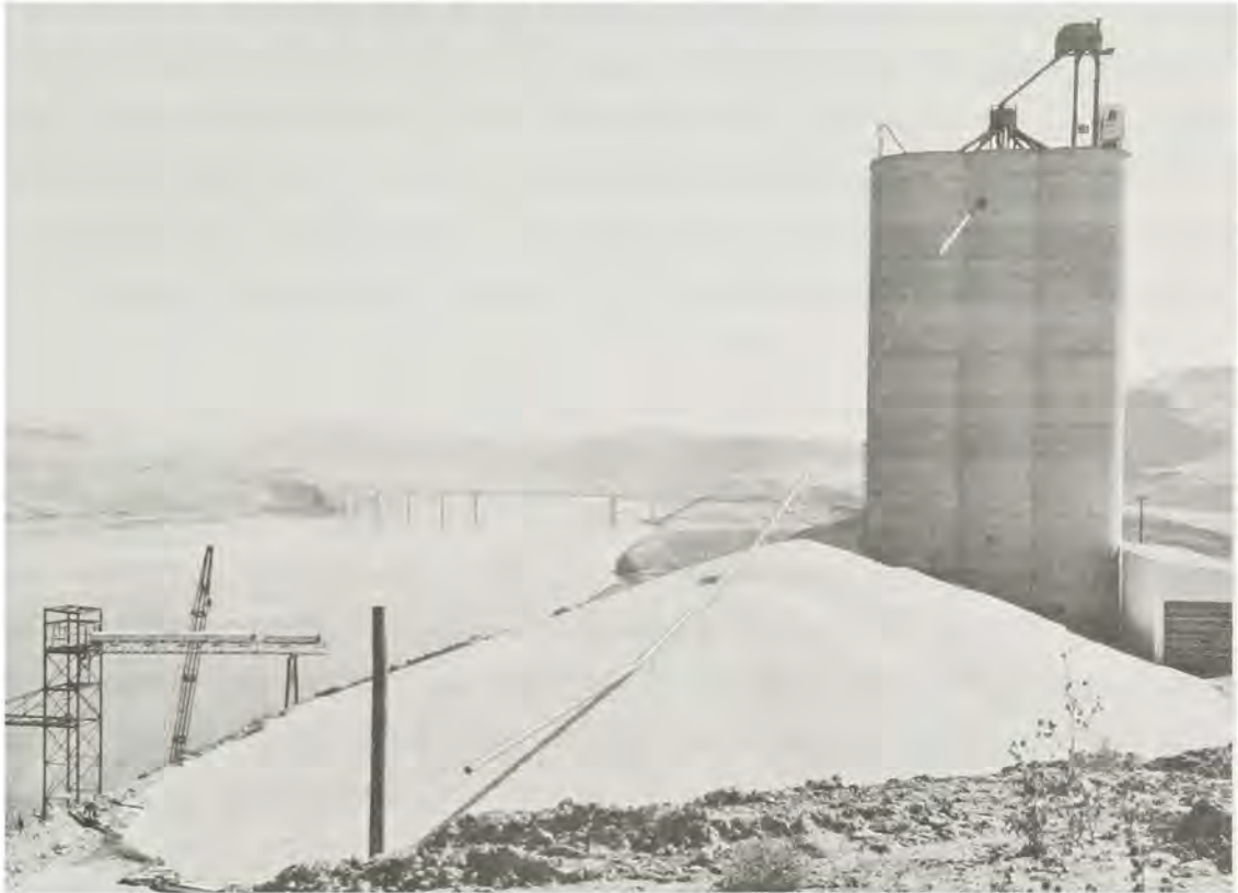
PORT OF COLUMBIA GRAIN ELEVATOR
