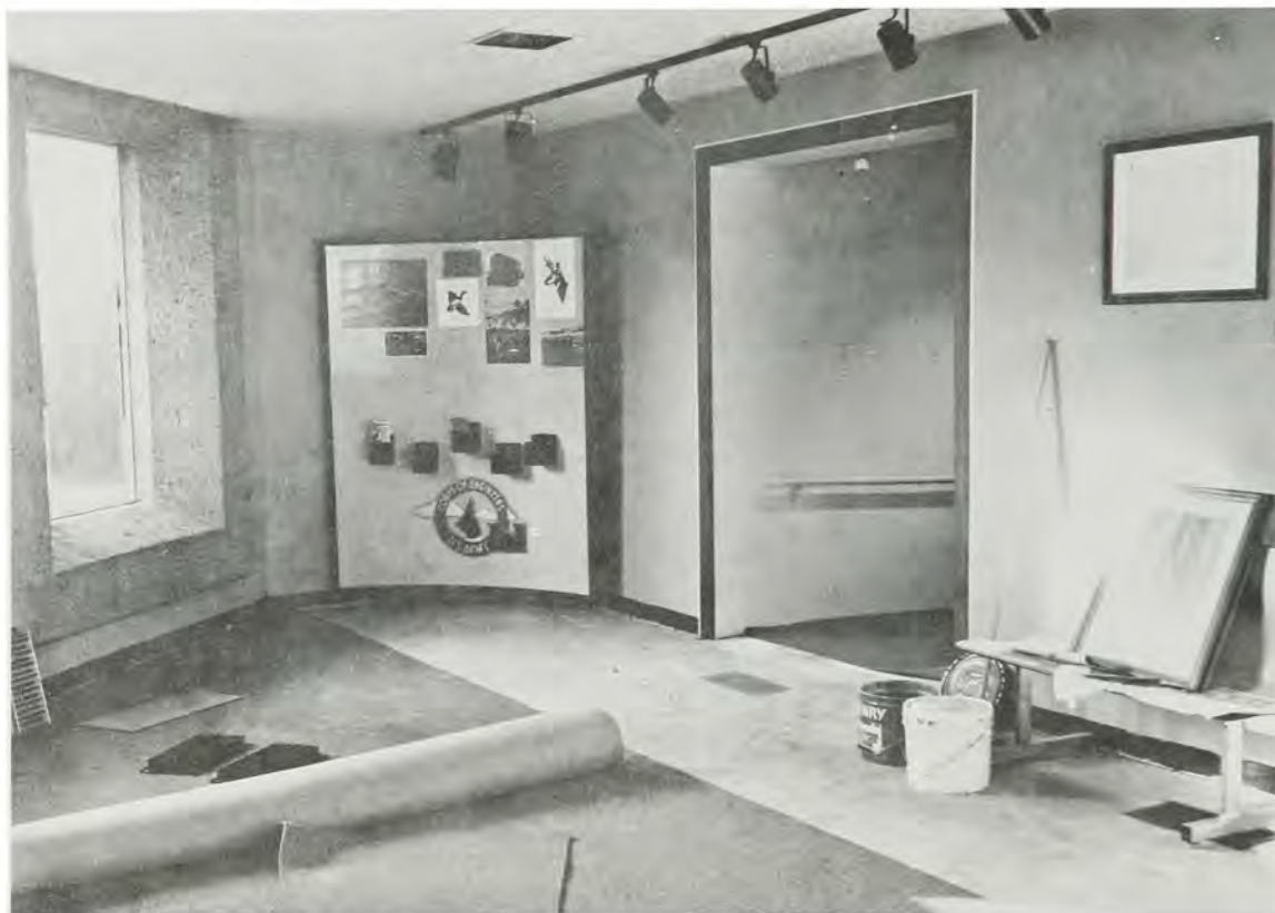
FISH VIEWING ROOM, ICE HARBOR VISITORS' CENTER UNDER CONSTRUCTION
