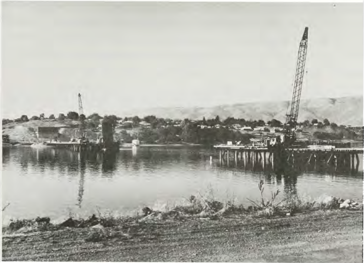
LEWISTON-CLARKSTON INTERSTATE BRIDGE UNDER CONSTRUCTION 1980
