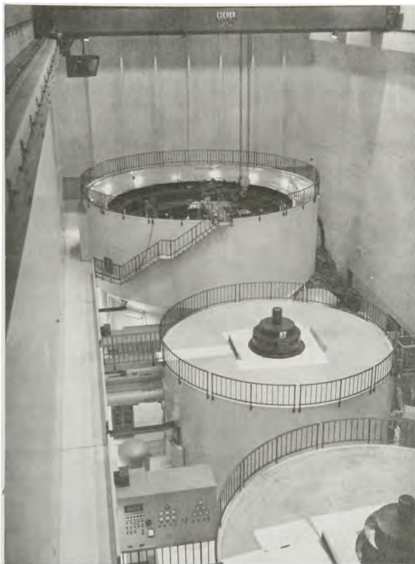
DWORSHAK DAM POWERHOUSE
