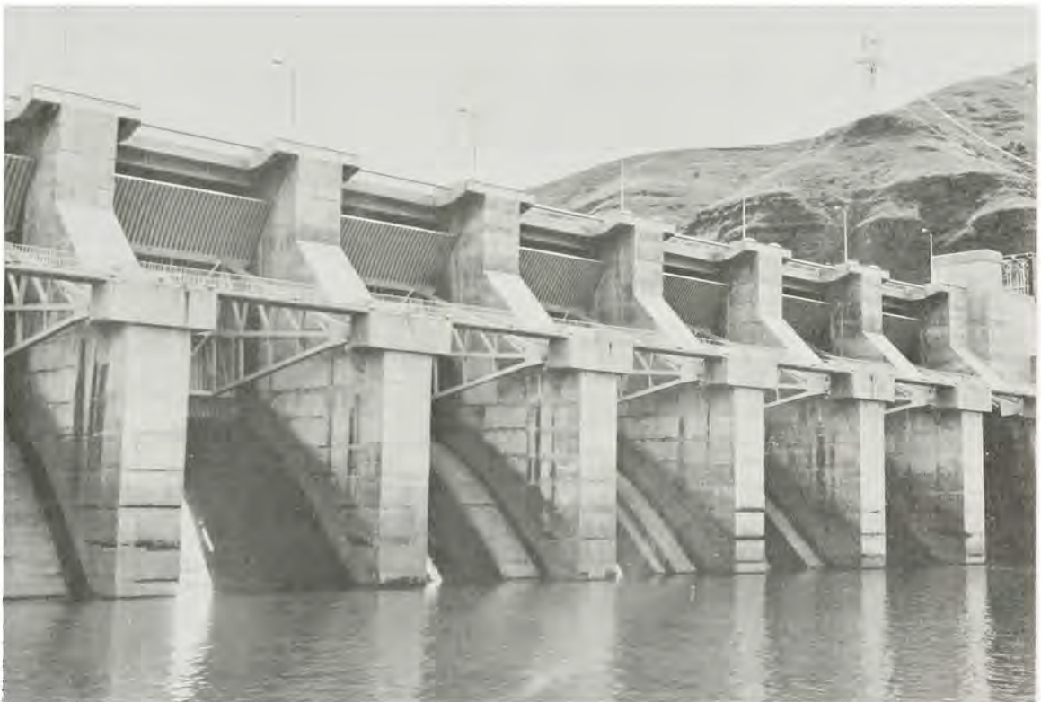
SPILLWAY BAYS LOWER GRANITE DAM
