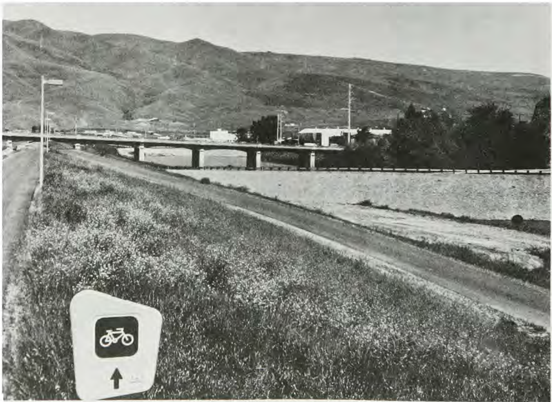
WEST LEWISTON LEVEE
