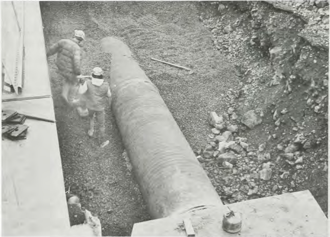
INSTALLING A FINGERLING BYPASS PIPE AT LITTLE GOOSE DAM
