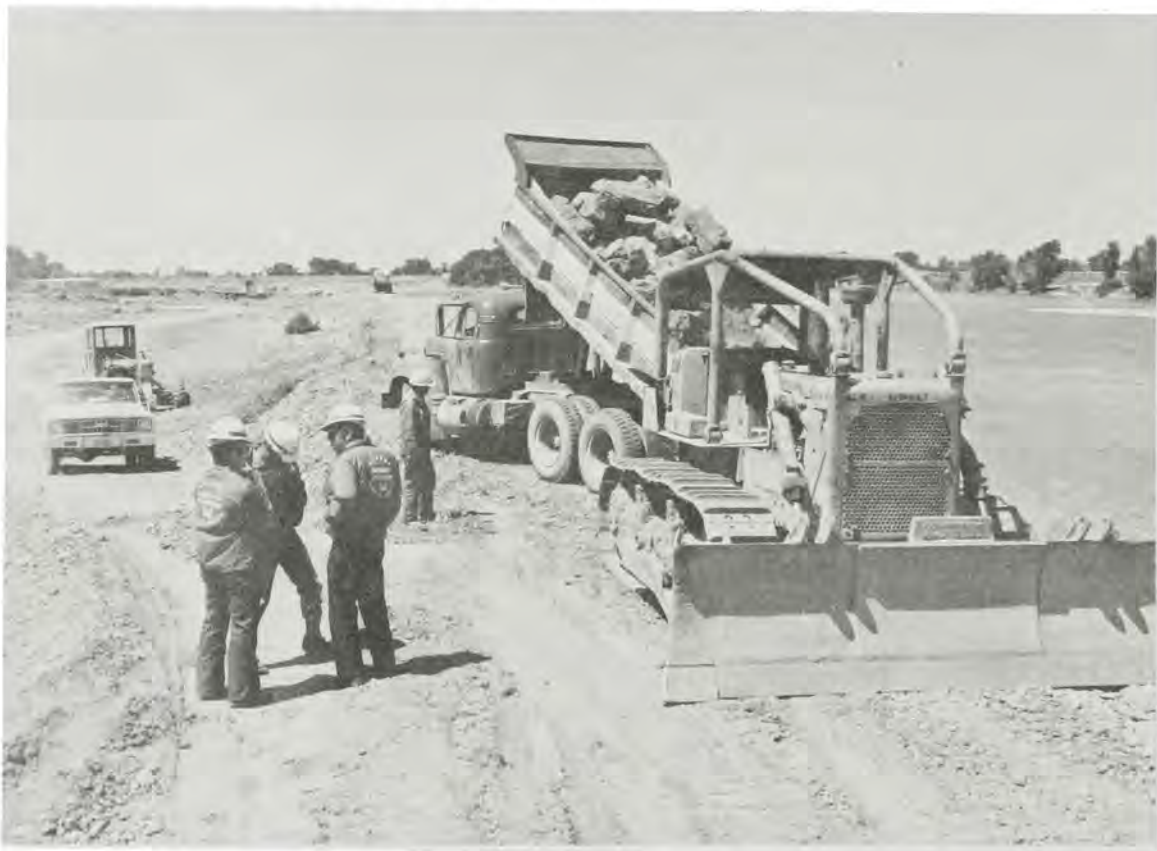
HANK VAN SCOTTER AND LIEUTENANT LANE GRIFFEN SUPERVISE LEVEE BUILDING
