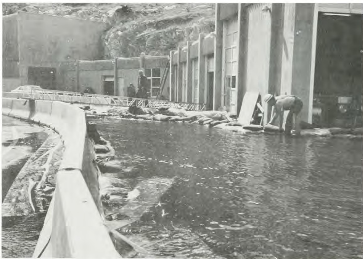
SANDBAGGING FOR TEMPORARY DIVERSION CANAL AT DWORSHAK
