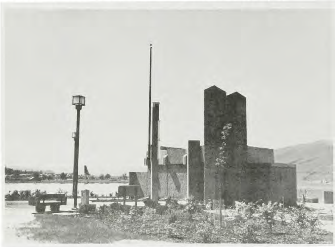
WEST LEWISTON LEVEE
