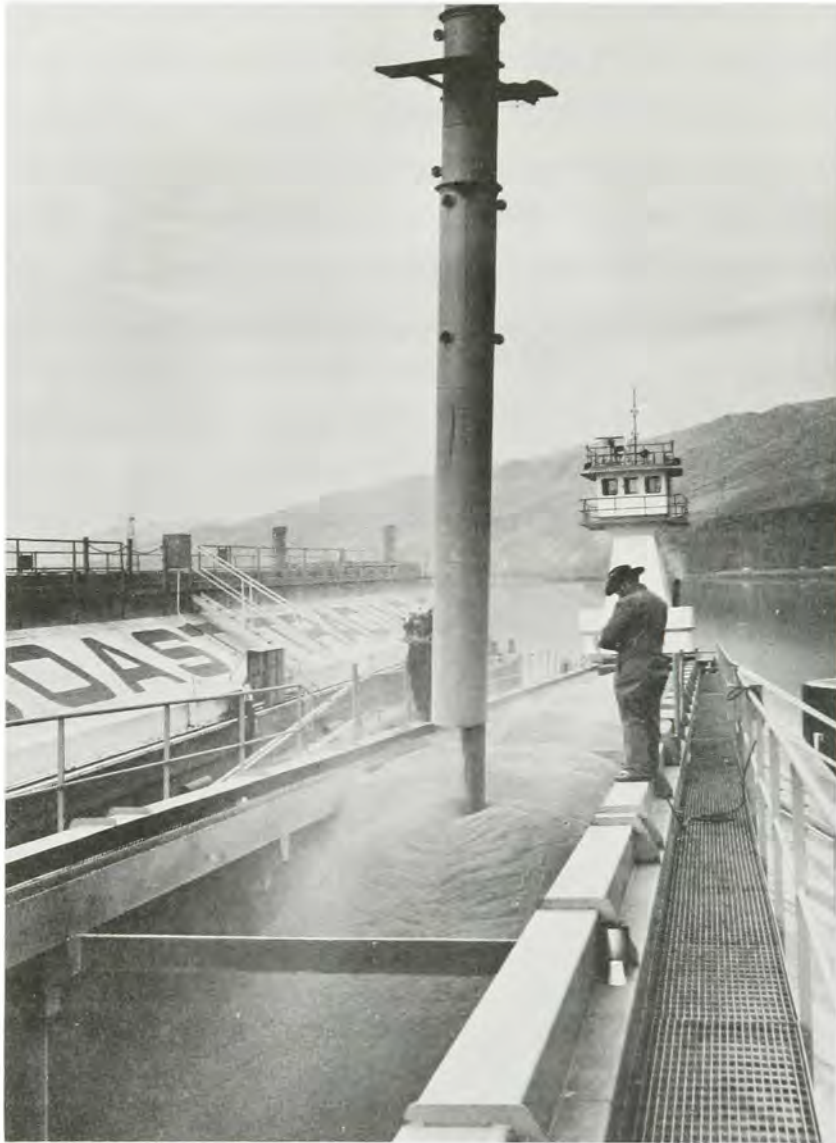
FILLING BARGE WITH WHEAT LOWER GRANITE LOCK
