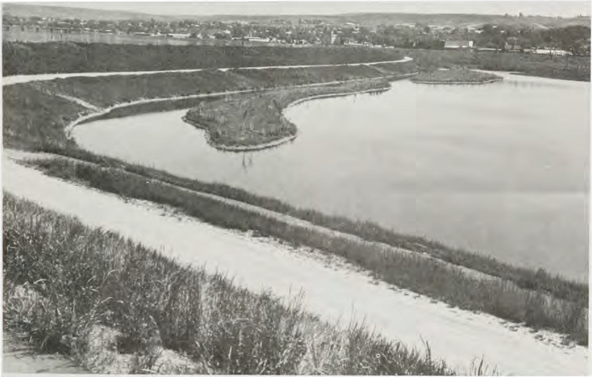
WEST LEWISTON LEVEE
