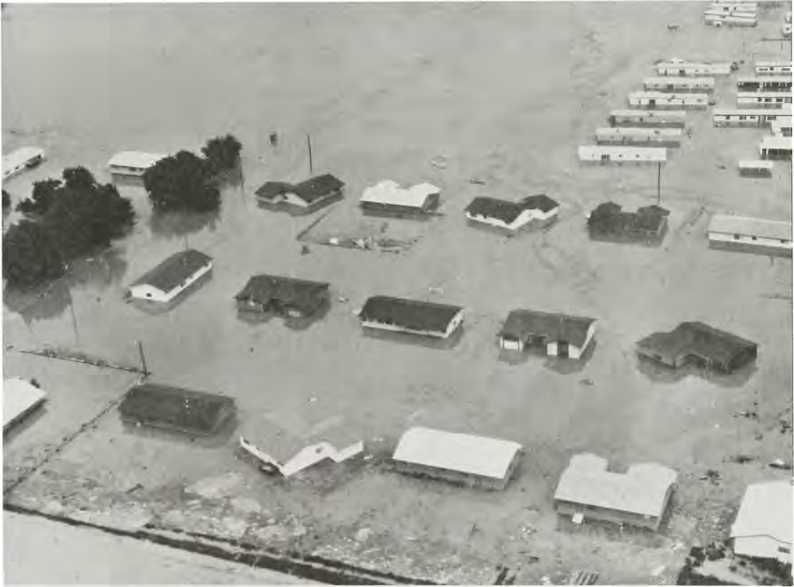
AERIAL VIEW OF FLOODING AT BLACKFOOT
