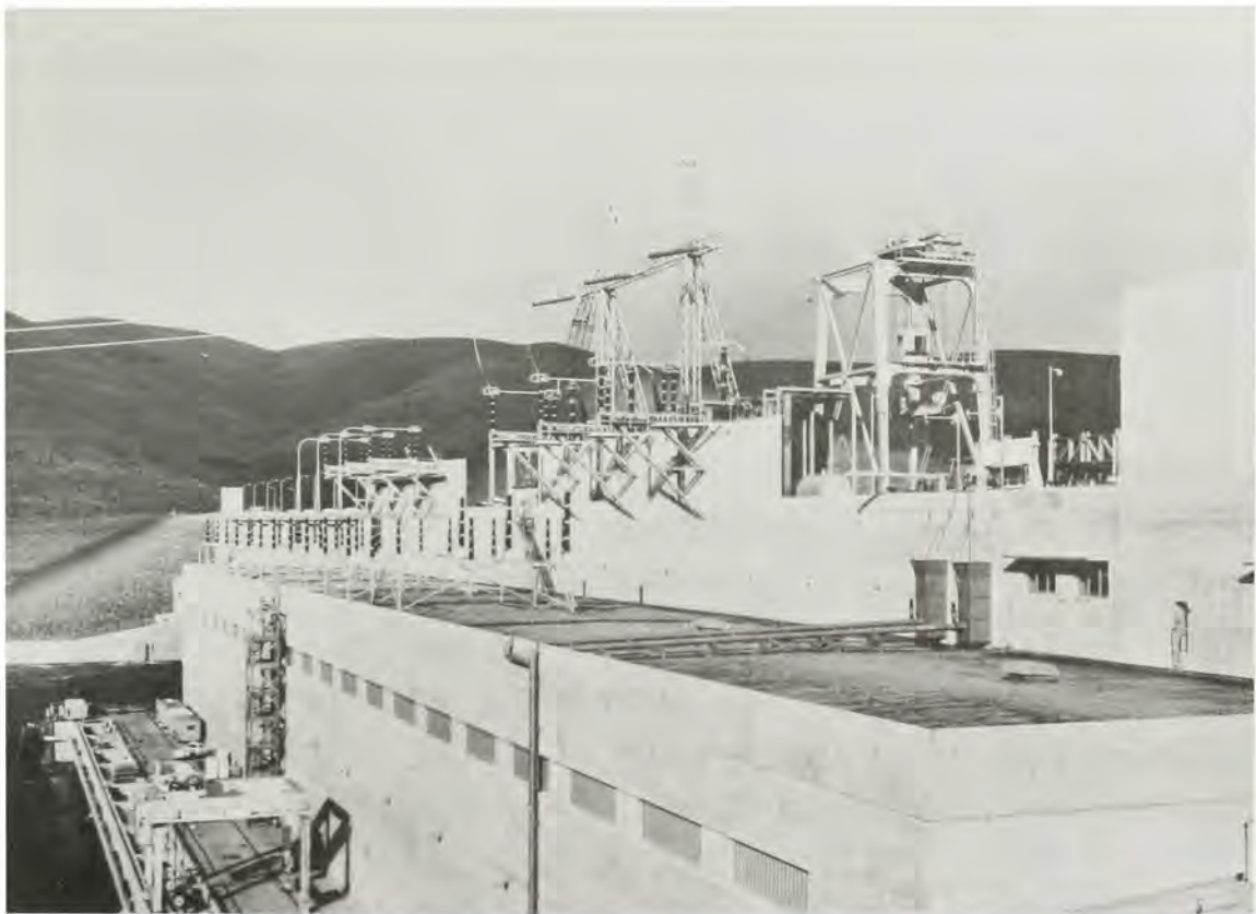
TRANSMISSION EQUIPMENT ON POWERHOUSE ROOF AT LITTLE GOOSE DAM
