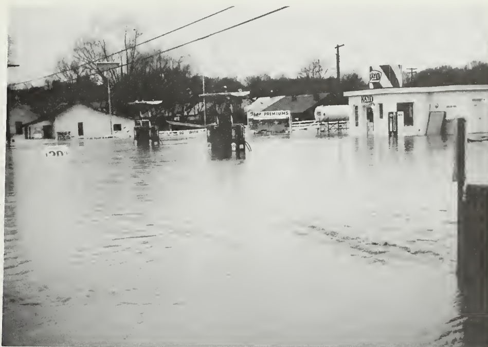
Flooding of commercial and residential property in Sweetwater along Vonore-Sweetwater County road in February 1961.
