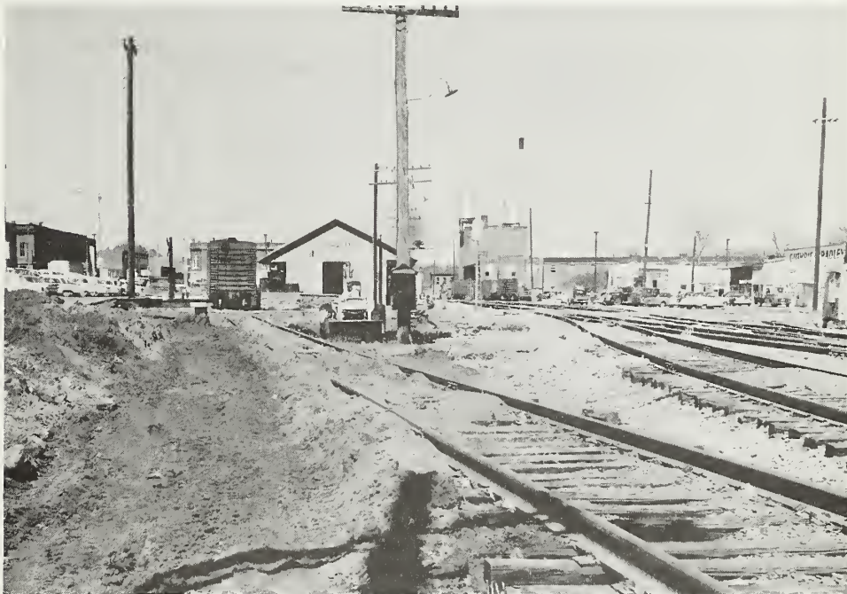
Sediment and erosion damage to main business district of Sweetwater and Southern Railroad from flooding of Sweetwater Creek on March 12, 1963.
