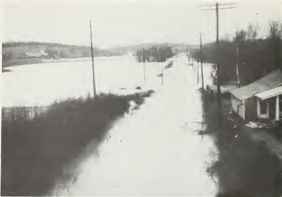
Southern Railroad and farm land covered by floodwater from Sweetwater Creek as viewed from U. S. Hwy. 11 looking south toward VS-56 and Sweetwater.
