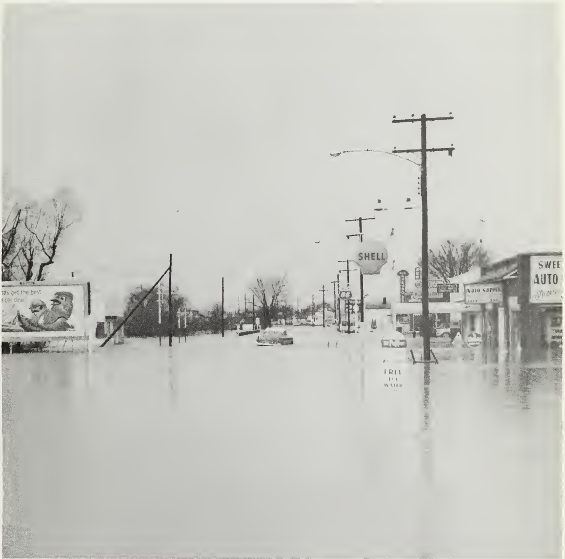
View of U. S. Highway 11 showing approach to the main business district, city of Sweetwater, from the south. About 30 inches of floodwater inundated road, Richesion Farm and Home Center, Sweetwater Auto Supply Company, and other commercial and residential property on March 12, 1963.
