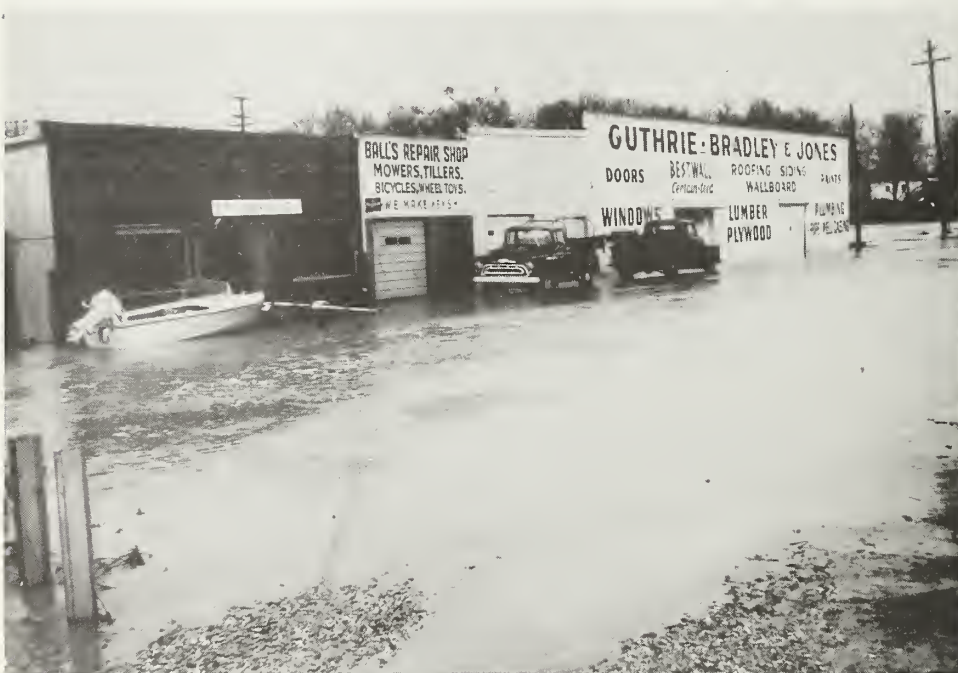
Commercial property damaged March 12, 1963 in Sweetwater as 24 inches of rampaging floodwaters inundated these buildings.
