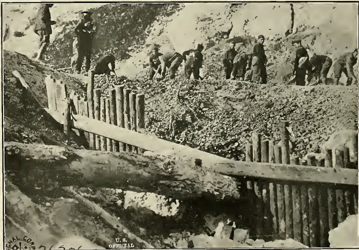
ENGINEERS REPAIRING ROAD
