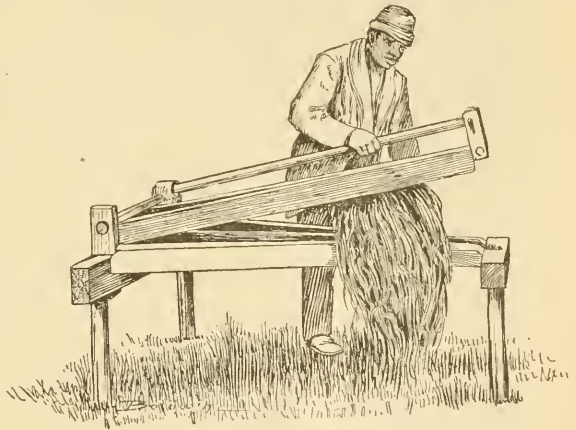
FIG. 38.—Kentucky hemp brake.
