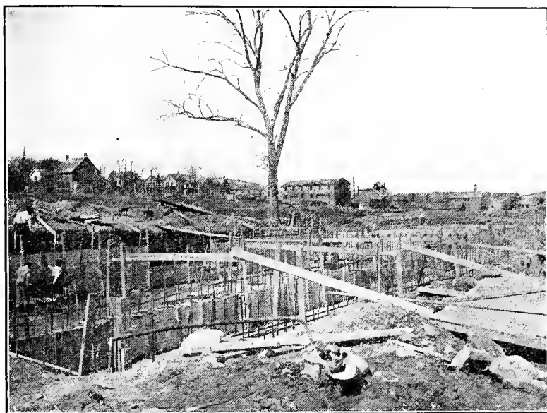
Showing the Settling Tanks During Construction.
