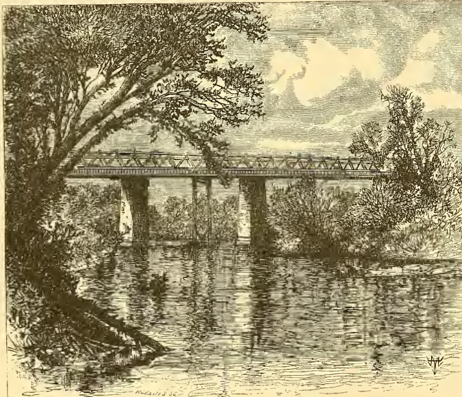
Bridge over the Marmiton River, near Fort Scott.
