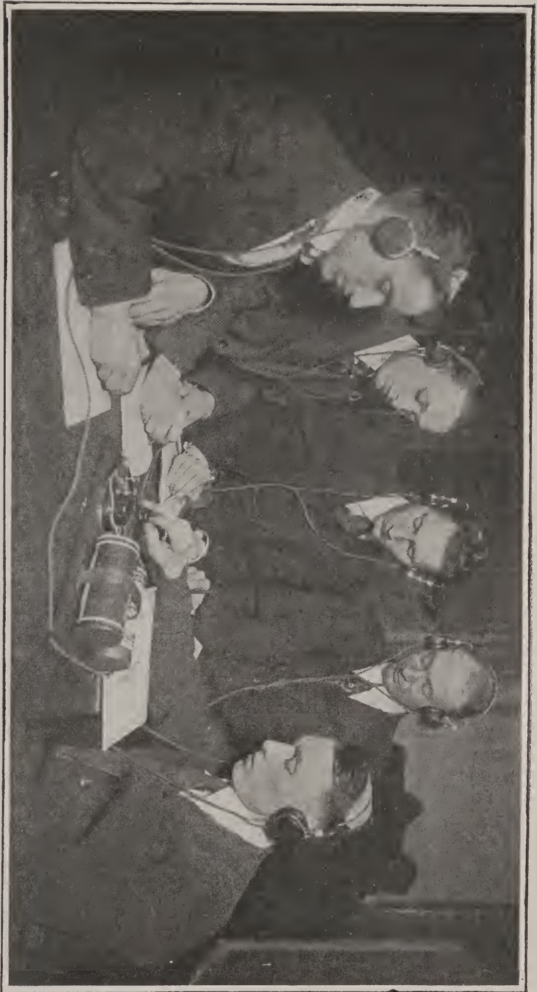
A group of young men learning the radio code. A telegraph key, high-pitch buzzer, and a couple of dry cells serve to simulate radio signals in the telephone receivers worn by the students and the instructor. The instructor sends out the messages, which are copied down by the students. At first the messages are simple and are sent at a slow rate of speed, but by degrees the speed is increased and the messages become more involved
