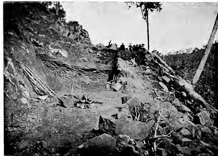
Work on the Railway—Blasting Rock
