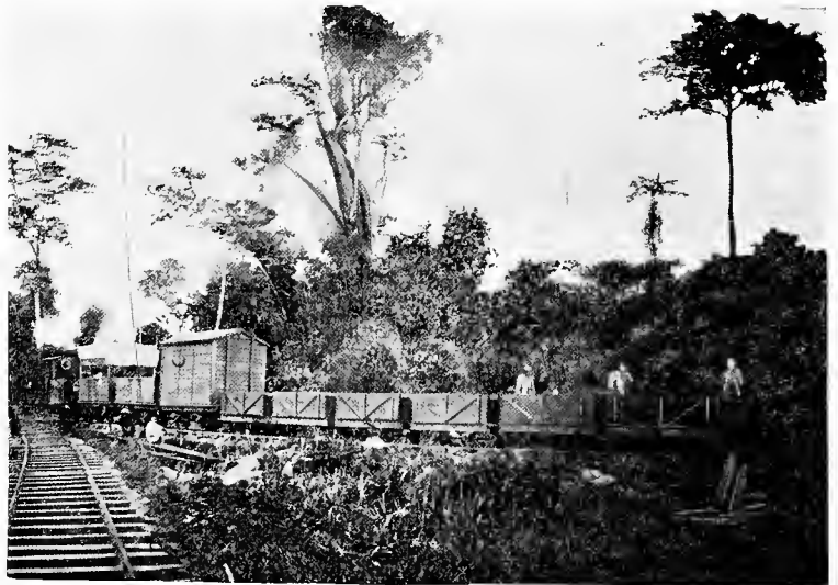
Railway Siding at Beaufort.
