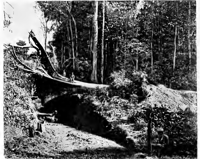
Fallen Tree across the Railway Cutting.
