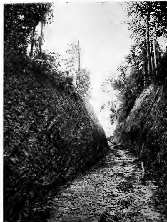
Railway Cutting on the Padas River
