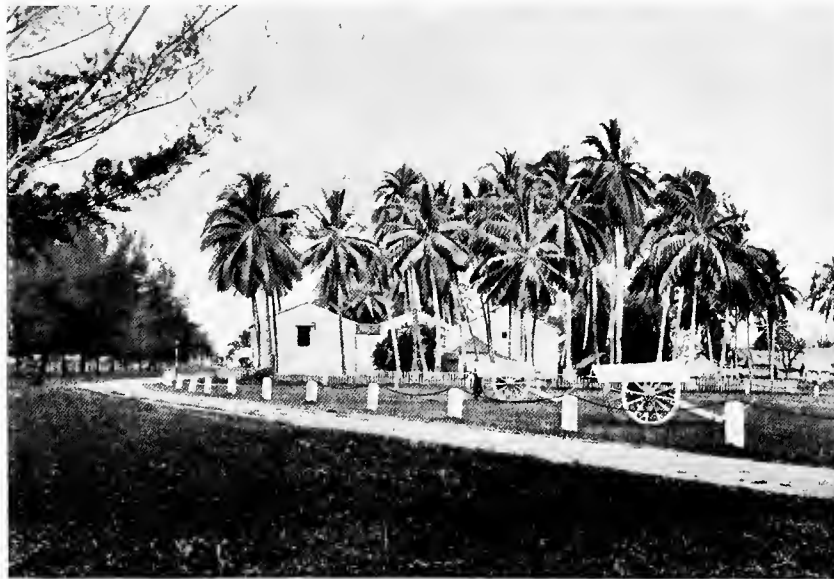
Road in front of Government Offices Labuan
