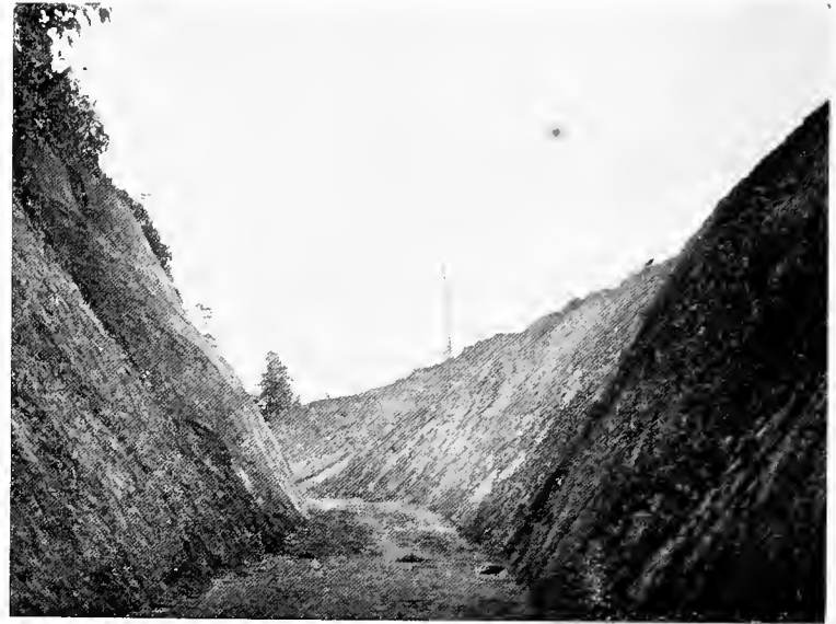
Railway Cutting on the Padas River.
