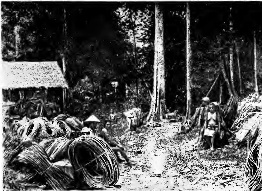
On the Route of Railway, Natives bringing down Jungle Produce.
