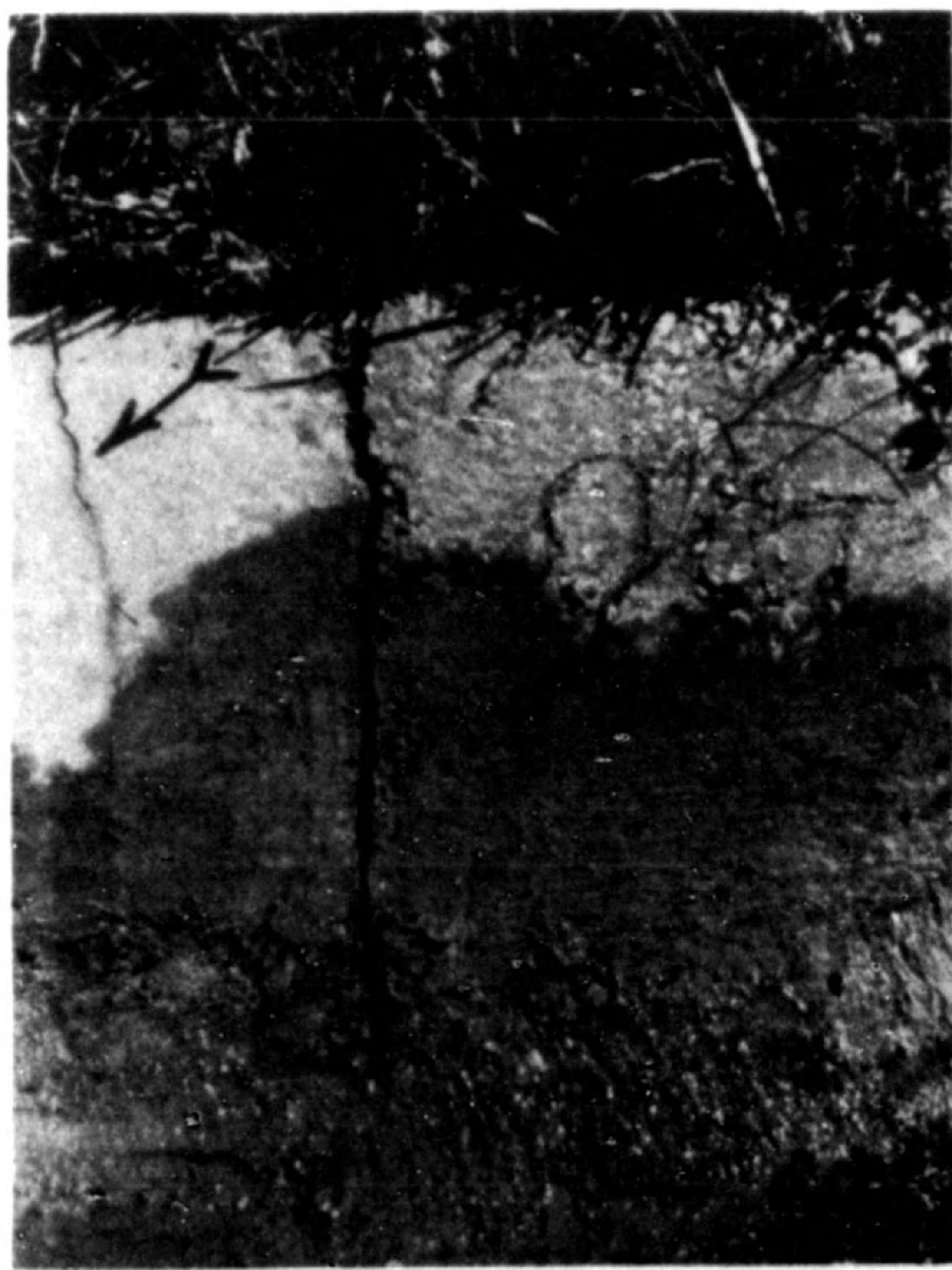
FIGURE 4.—Crack at extreme left (arrow) caused by compression resulting from lack of expansion joint between the two sections. Dark line along ends of slabs (center) is not an opening but a shadow cast by slab on right which has "overlapped" slab on left.
