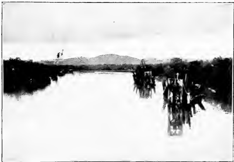
FRENCH DREDGES SUNK IN RIO GRANDE.
