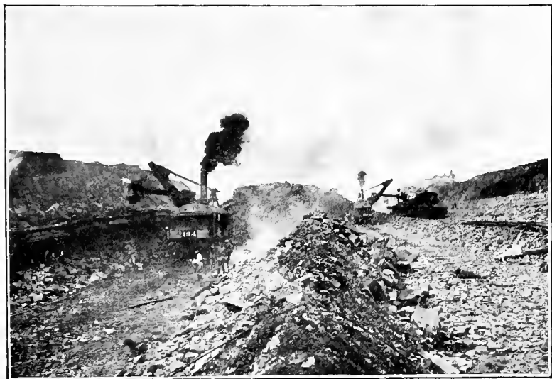
EXCAVATING FOR GATUN LOCKS.
