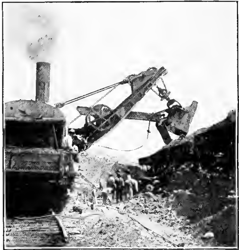
STEAM SHOVEL—SHOWING ARM AND DIPPER.
