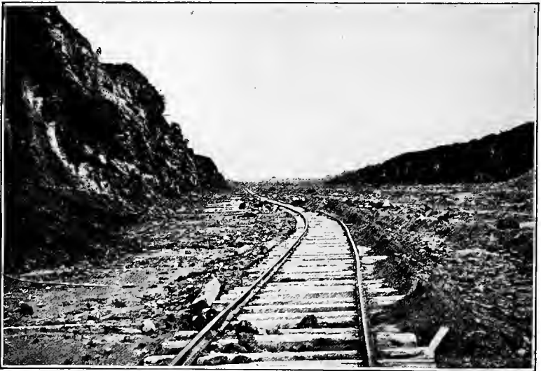
EXCAVATION FOR GATUN LOCKS COMPLETED.
