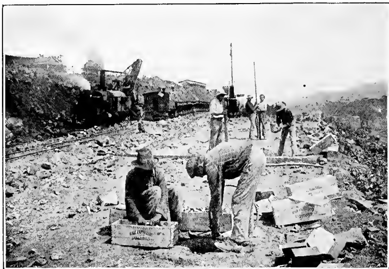
LOADING DRILL HOLES WITH DYNAMITE.
