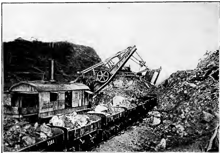
LOADING DIRT TRAIN BY STEAM SHOVEL.
