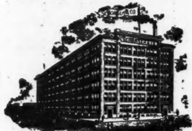
FACTORY 132 ND TO 133 RD ST. & BROOK AVE
