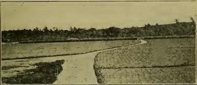
Fig. 118.—Cranberry bog newly planted, showing ditch and dike; also portion of bed not yet covered with sand.
