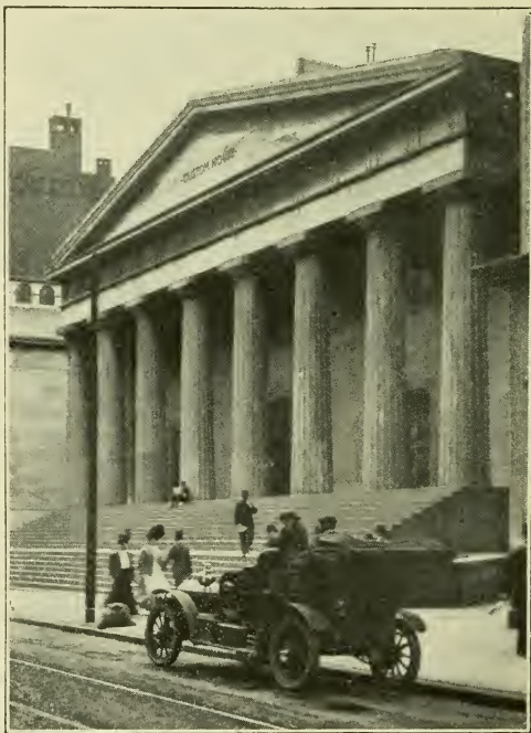
U. S. Custom House Chestnut between S. 4th and S. 5th Streets Page 56
