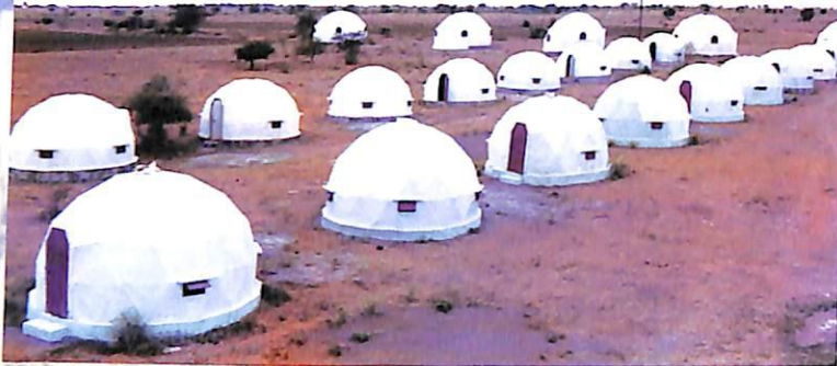
Pabal dome constructed in earthquake rehabilitated village
