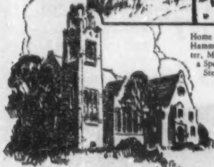
Lake Avenue Baptist Church, Rochester, N. Y. Two Spencer Heaters are adequate to heat this building in severest weather.
