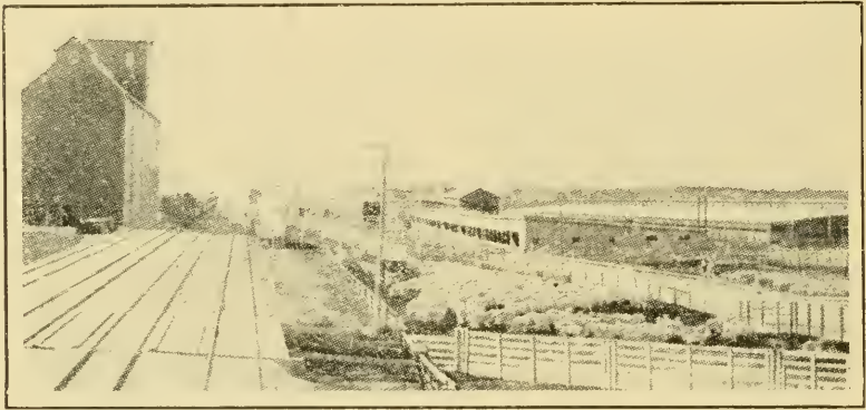
AN ILLINOIS FEEDING AND SHIPPING YARD.
