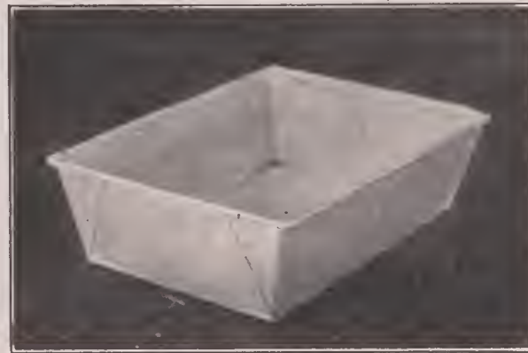
Problem 103. Rectangular Flaring Pan with Folded Corners.
