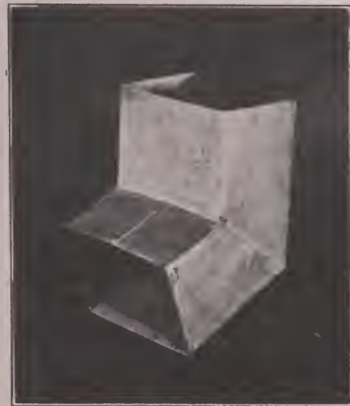
Problem 3. Rectangular Conductor Shoe.
