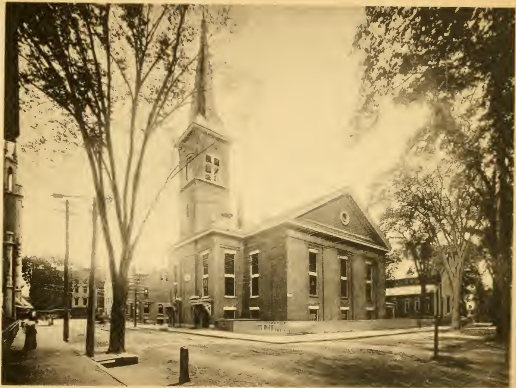
FRANKLIN STREET CHURCH.
