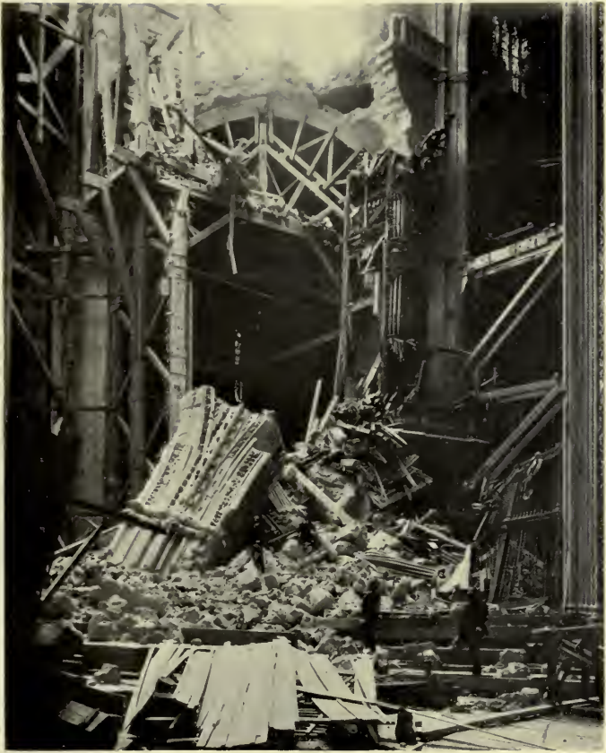
COLLAPSE OF THE CENTRAL VAULTS, SEVILLE CATHEDRAL.
