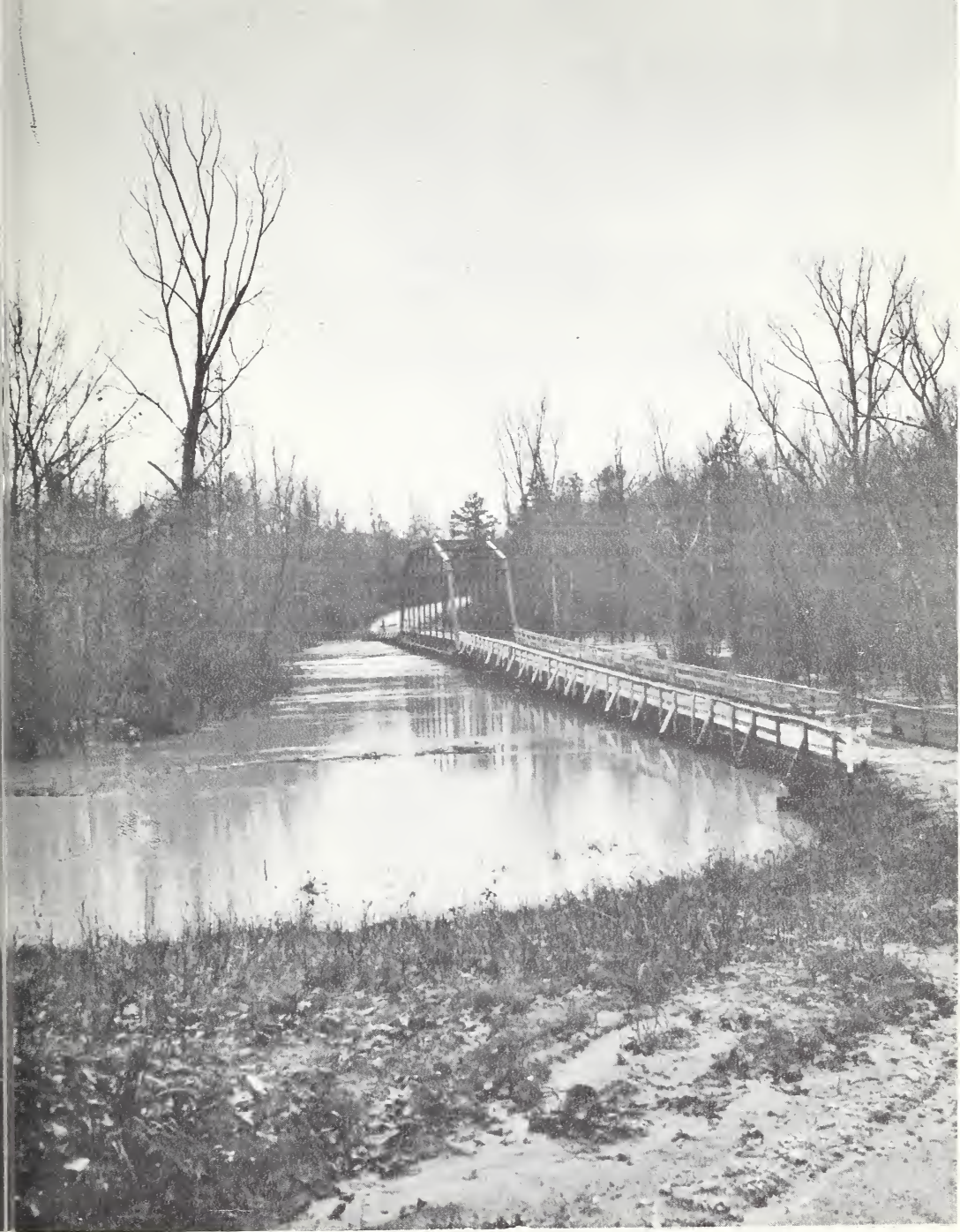
Figure 12.—Bridges in the Piedmont have to span the flood plain as well as the river.
