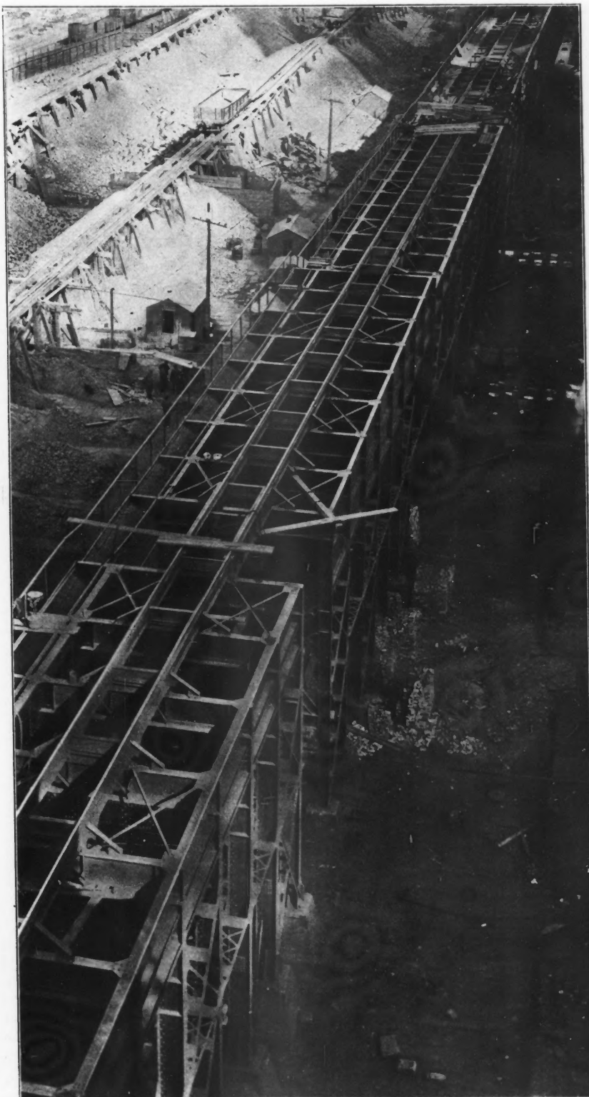
BINS FOR ORE, COKE AND LIMESTONE AT MINNEQUA WORKS
