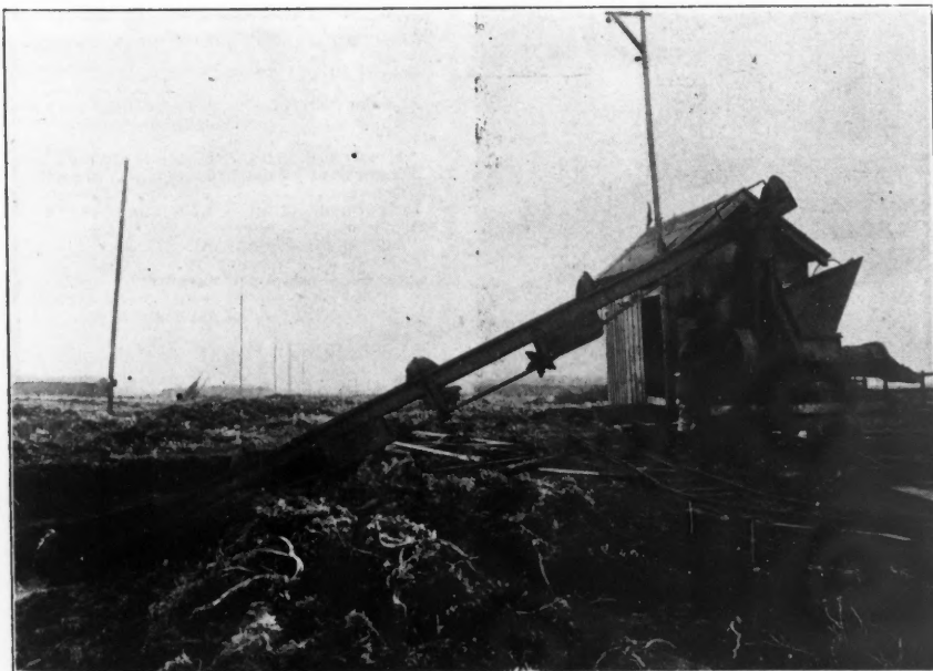
FIG. 1. PEAT MACHINE. IN THE BACKGROUND ARE HEAPS OF AIR-DRIED PEAT
