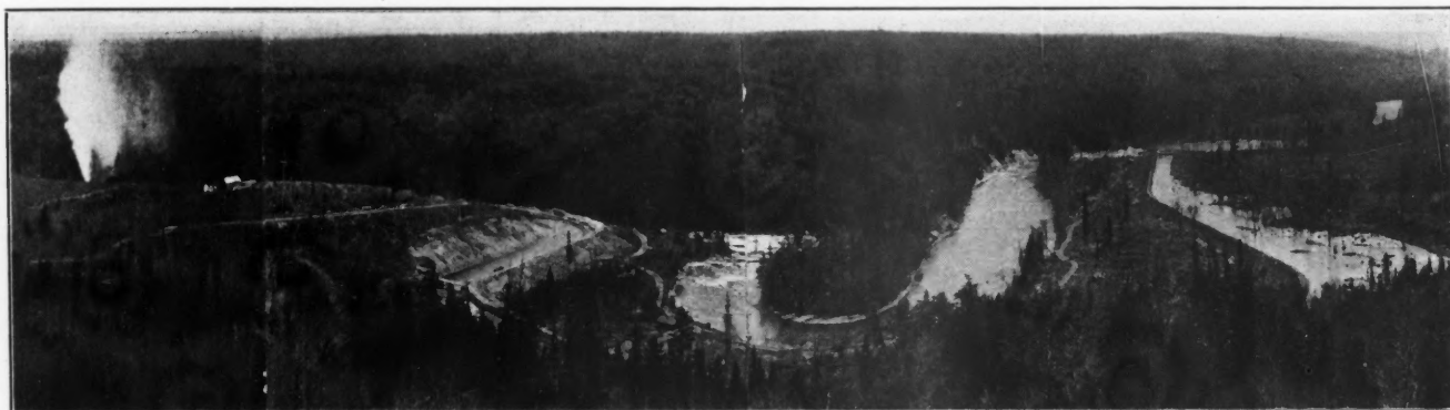
VIEW OF THE DAM, A PORTION OF THE CANAL, THE COMPRESSOR HOUSE AND THE BLOW-OFF
