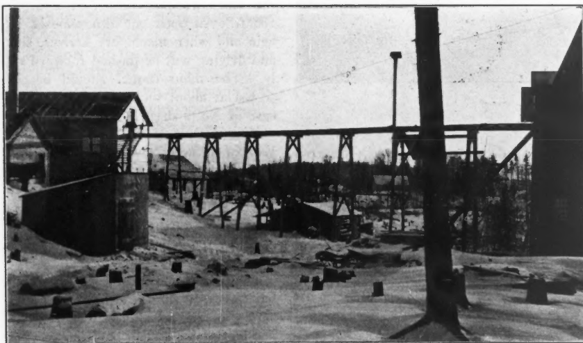
ORE-HOUSE, TRESTLE AND SHAFT AT CONIAGAS MINE
