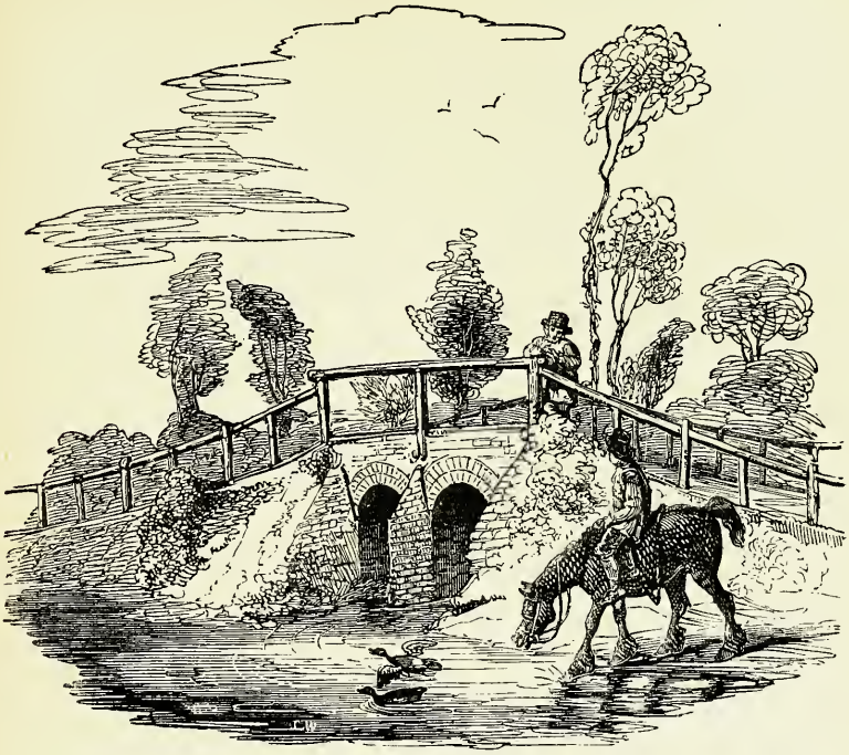
BRIDGE ON THE ROAD TO BECKENHAM.
