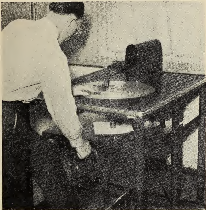
FIGURE 11.—Improved templet cutter. This machine can be set automatically to change scale between photographs and templets.
