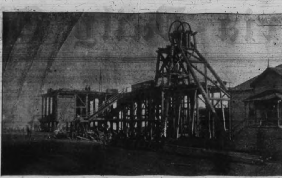
NEW VANCOUVER COAL CO. NO. 1 SHAFT.
