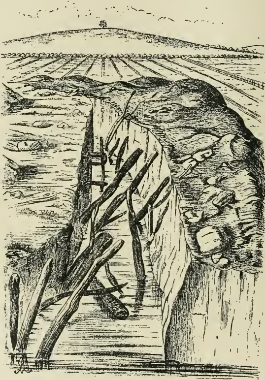
Fig. 34.—View of the Trench on the North side.
