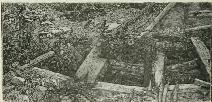
Fig. 190.—Portion of north side of Crannog, with the space between inner and second circle of piles dug out, showing arrangement of Transverse Beams and structure of the Log Pavement. ( From Photograph by Mr. Laurie. )
