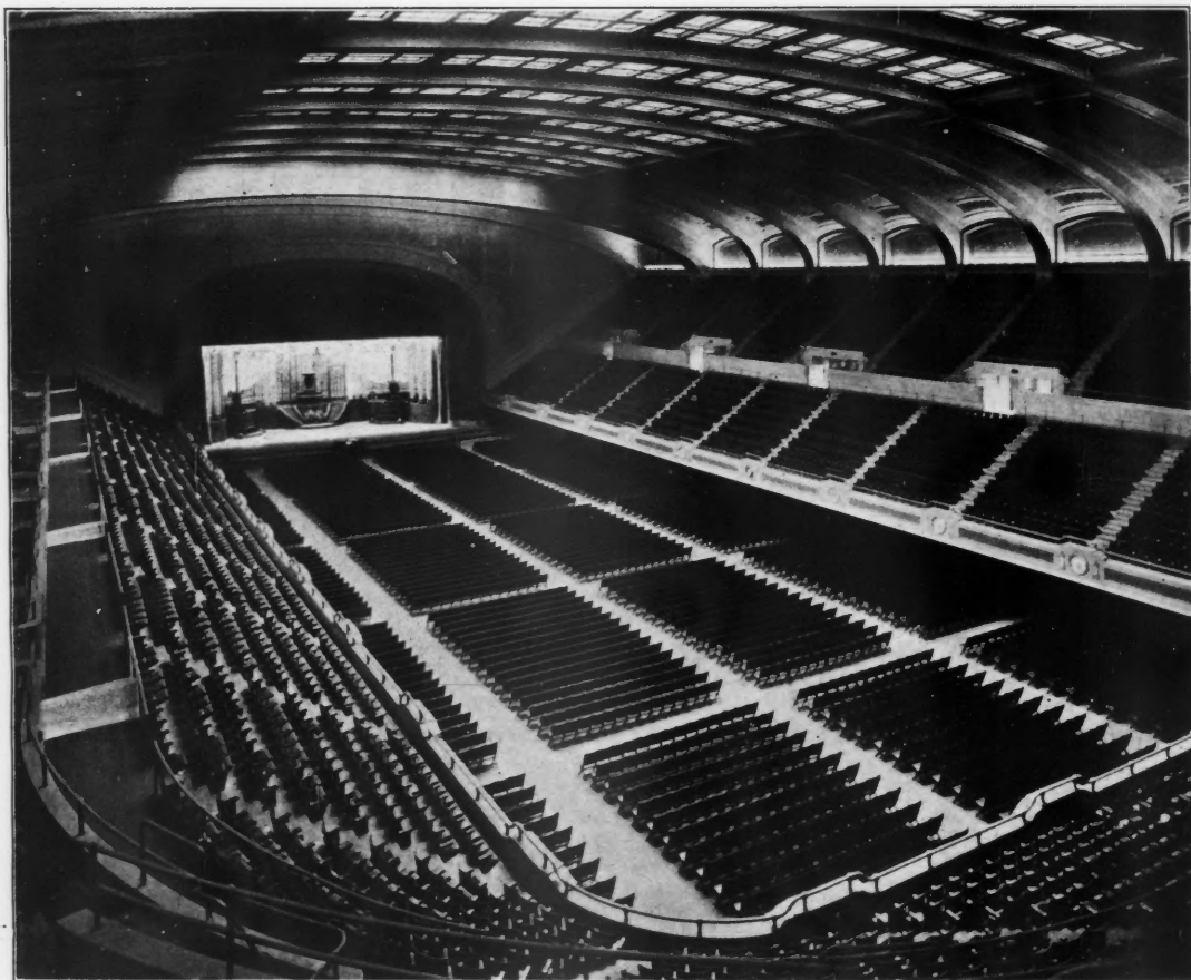
Cleveland's gigantic new convention hall, where 578 reporters will serve as eyes for the nation when the Republicans meet to nominate their party's choice for President. Under the stage, in the background, it is planned to locate the workrooms for the press and telegraph services. Reporters will be seated on both sides of a runway to be constructed from the stage down the middle aisle.
