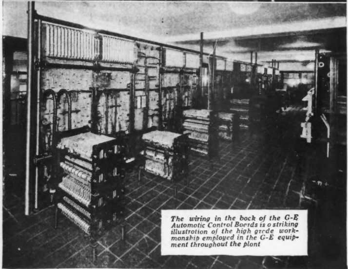
G-E Automatic Electric Control Boards which operate the press so smoothly through all of its functions, are located in a glass-enclosed mezzanine gallery
