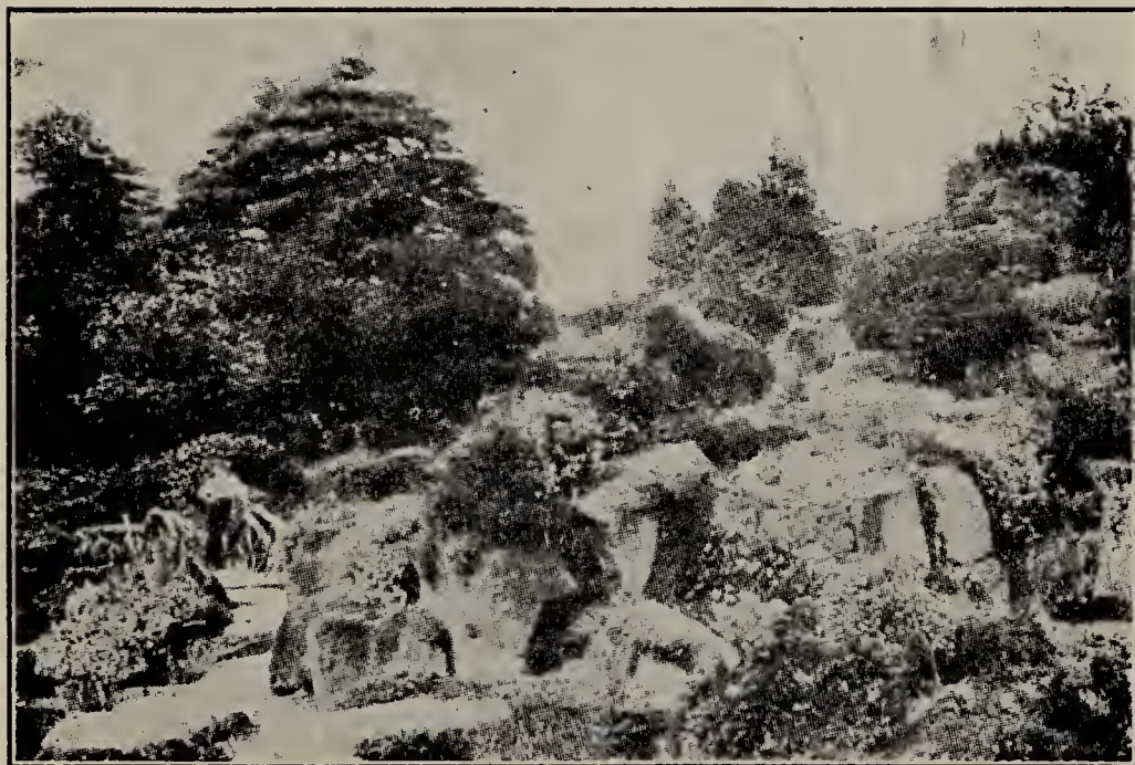
Construction of the Rockery
