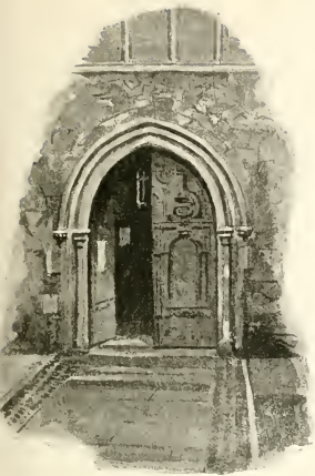
DOOR, ST. HELEN'S CHURCH, BISHOPSGATE STREET
