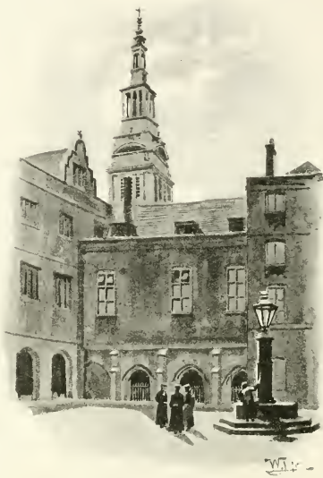
CHRIST'S HOSPITAL, CLOISTER
