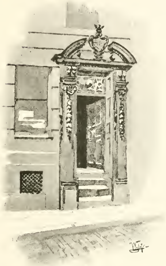
PAINTERS' HALL, ENTRANCE
