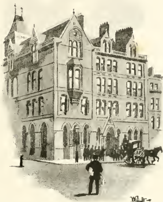
PRUDENTIAL ASSURANCE COMPANY'S OFFICES IN HOLBORN
