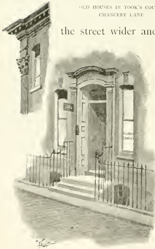
DOORWAY IN TOOK'S COURT, CHANCERY LANE
