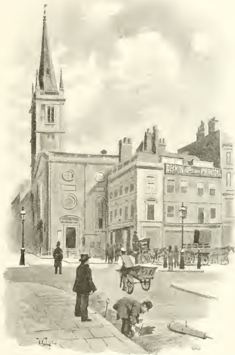
ST. MARGARET'S CHURCH AND OLD HOUSES IN EASTCHEAP
