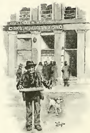
EIVES AND ALLEN'S OFFICES (AGENTS OF THE INMAN LINE AND WELLS FARGO'S EXPRESS), 99 CANNON STREET, E.C.
