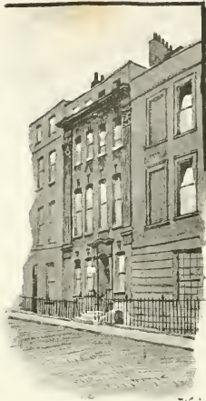
OLD HOUSES IN TOOK'S COURT, CHANCERY LANE
