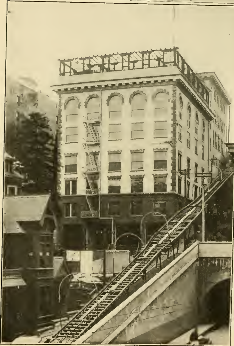
LOOKING FROM HILL STREET
