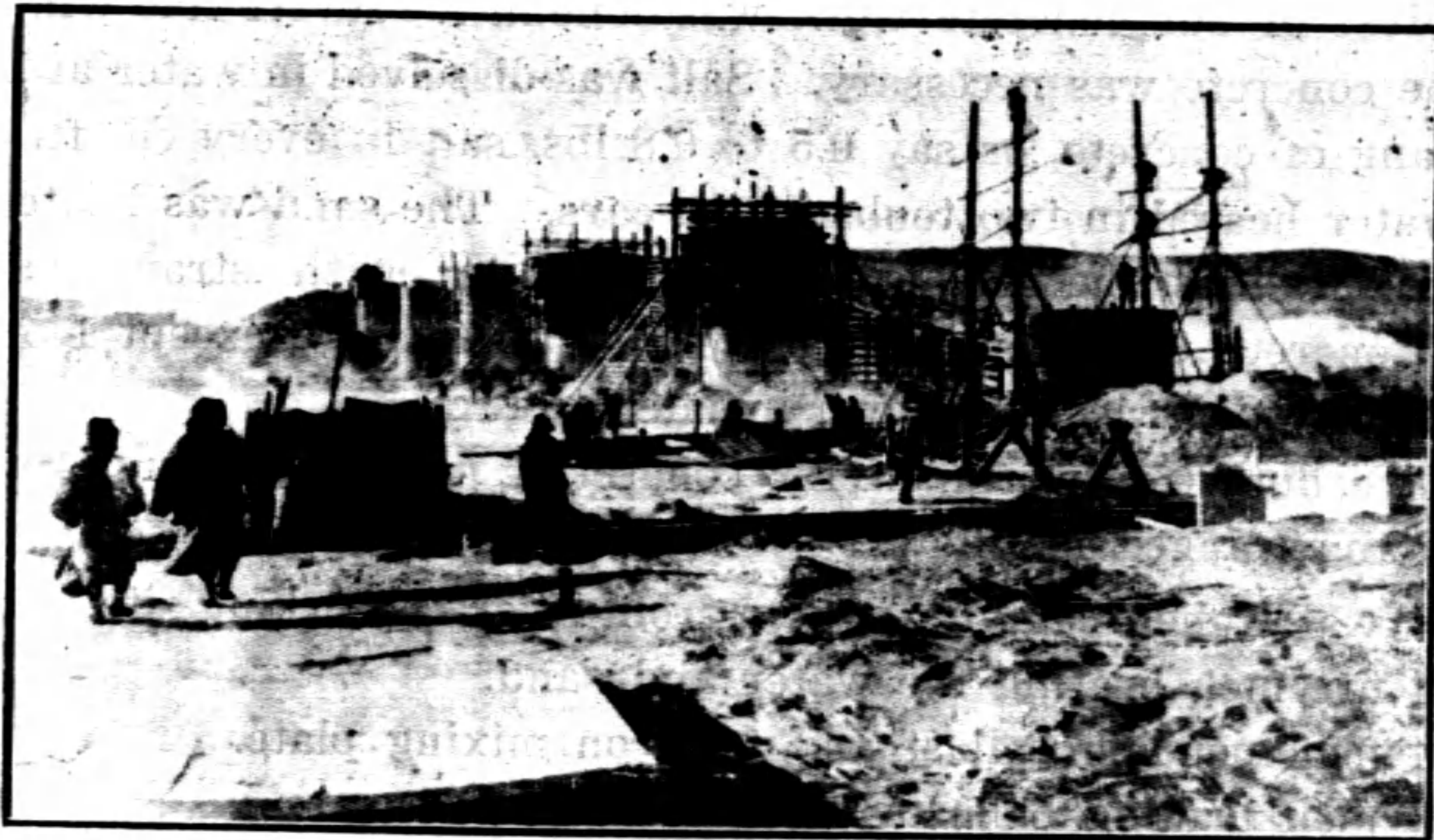
(H) Scaffolding to Pier Moulds (Courtesy of Mr. Y. Y. Wu)
