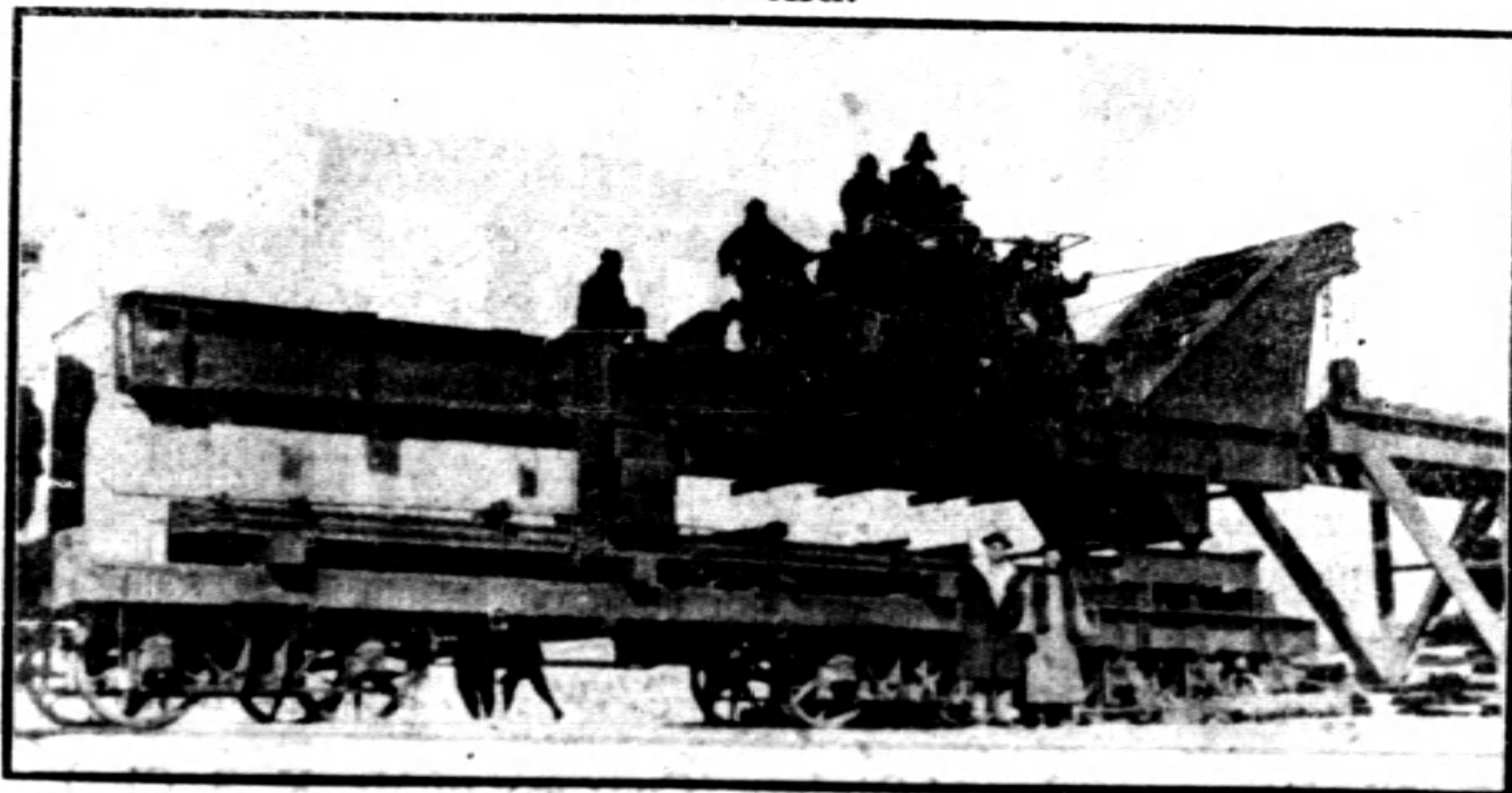
(K) The Girder-Erection-Crane (Courtesy of Mr. K. S. Chu)
