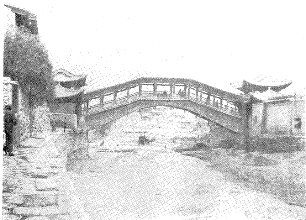
△ Hatching Bridge, Lanchow
