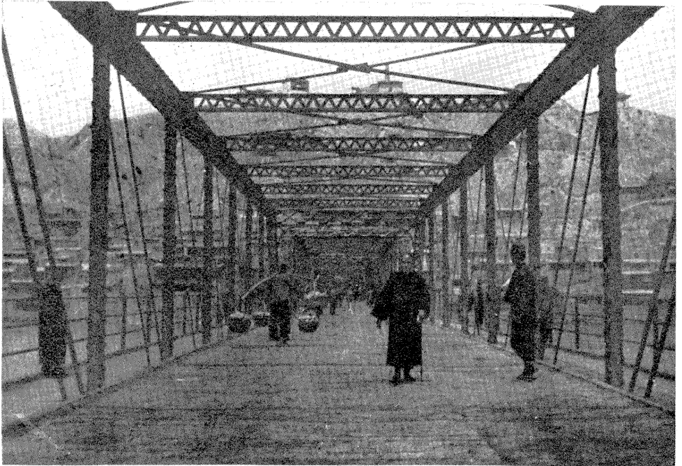
Views of Yellow River Bridge, Lanchow
