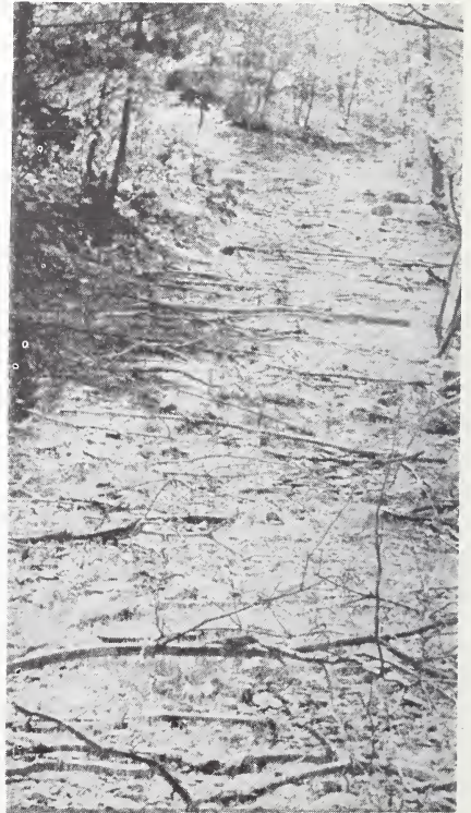
Figure 32 — Erosion on logging roads can be controlled. Before and after pictures of an eroding skidroad to which simple protective measures have been applied. Grade is about 25%.
