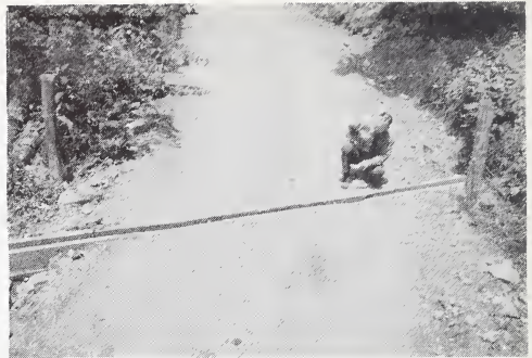
Figure 10 — Open-top box culvert properly installed in road.
