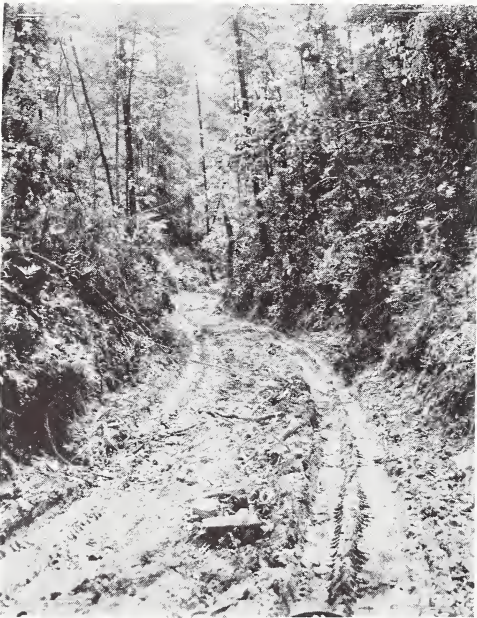
Figure 2—Poorly located logging road with no facilities for drainage.
