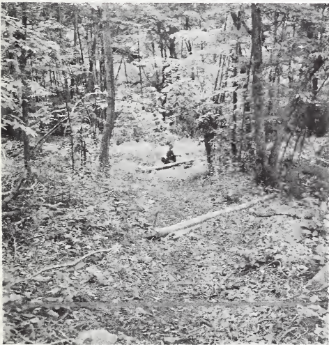
Figure 31 — Water bars installed in abandoned skid trail to prevent erosion.
