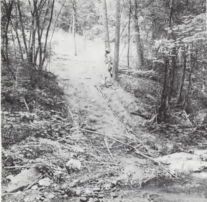
Figure 28 — Before this steep section of tractor road was seeded down it deposited much silt and debris in stream channel.
