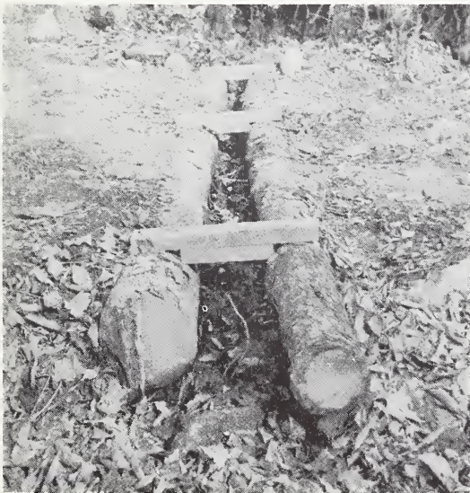
Figure 13 — Open-top pole culvert installed in logging road.
