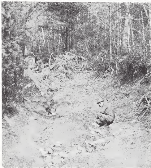
Figure 15 — Abandoned logging road in light soil now seriously eroding. Simple protective measures could have prevented this.
