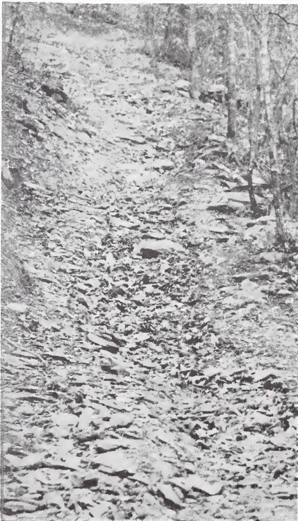
Figure 32 — Erosion on logging roads can be controlled. Before and after pictures of an eroding skidroad to which simple protective measures have been applied. Grade is about 25%.
