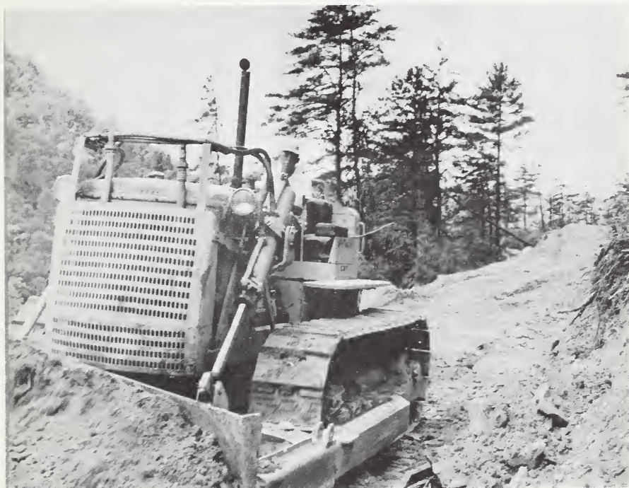
Figure 4 — Bulldozer at work on road construction.
