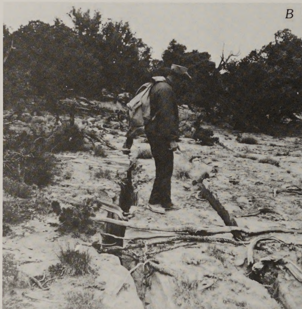
FIGURE 12.—Effects of underground coal mining on land subsidence. A , Generalized cross section showing subsidence and fracturing that occurs above an underground coal mine (modified from Lines and others, 1984). B , Fractures resulting from subsidence at the surface above a barrier pillar in an underground mine in Utah (from Lines and others, 1984).
