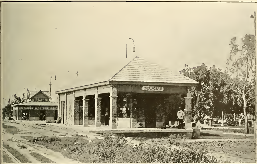
Railroad Station at "Delicias," Oriente Province
