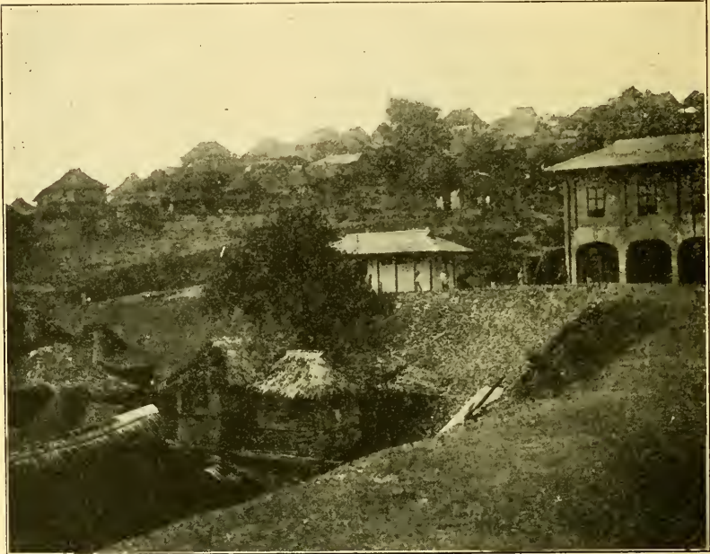
CONCRETE DORMITORY AND NATIVE SHACKS.
