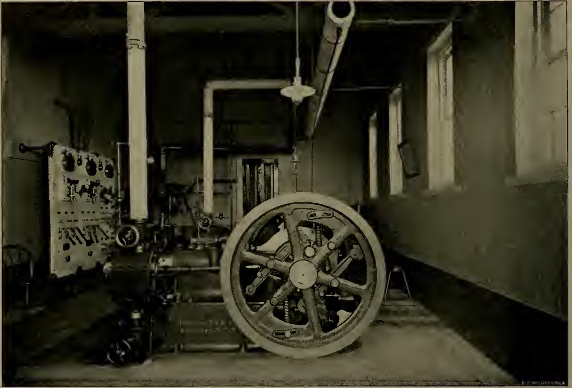
ELECTRIC PLANT - DYNAMO ROOM
