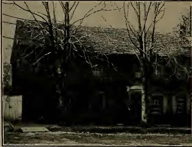
OLD STEPHEN ESSER HOUSE (FRONT VIEW) - DEMOLISHED
