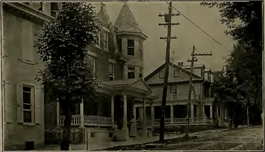
HANDSOME HOMES ON UPPER MAIN STREET (The stone house to the right is the remodeled First House Erected in "Freetown")
