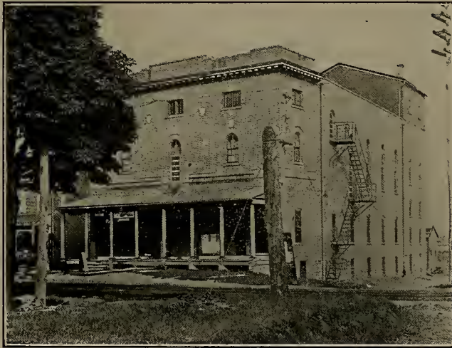
THE KUTZTOWN AUDITORIUM
