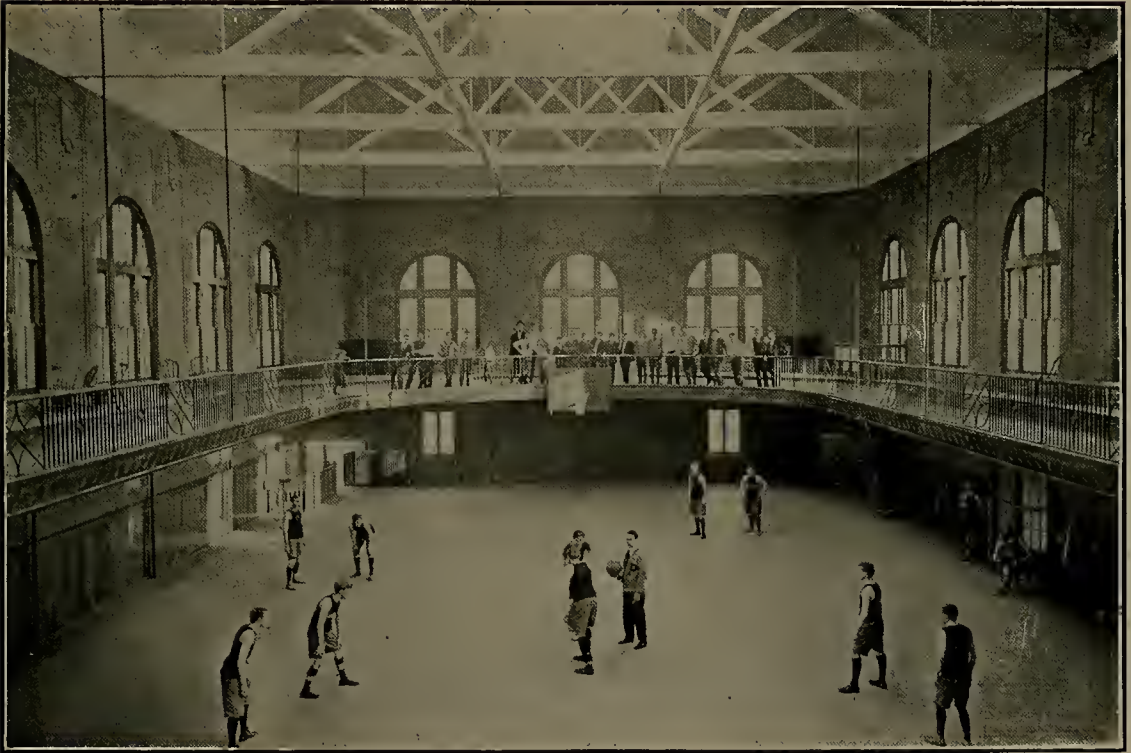
INTERIOR OF GYMNASIUM—BASKET BALL PRACTICE
