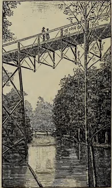
THE HIGH BRIDGE.
