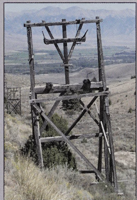
This tram tower from the early 1900s is part of an aerial tram system in the White Knob Mining District in southeast Idaho. The tram was used to move ore over 4 miles from the Empire Mine to the railroad.
