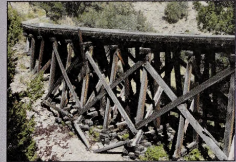
This historic railroad trestle in the White Knob Mining District is being restored as part of a recreation trail.
