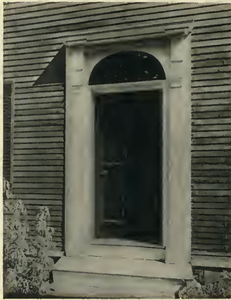
Detail of Entrance.
