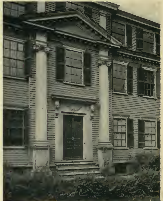
Detail of Entrance and Pediment.
