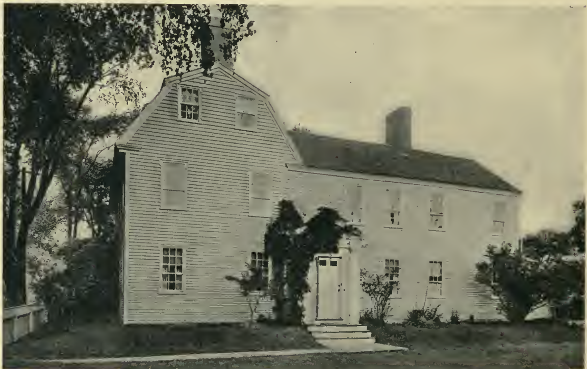
THE EMERY HOUSE AT NEWBURYPORT, MASSACHUSETTS. Built in 1796 by Thomas Coker, Architect. A good example of the New England gambrel roof type.
