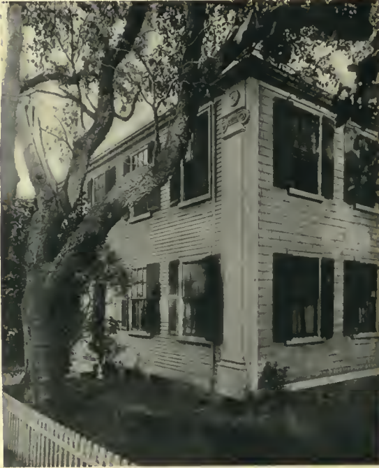
Detail of Pilaster.
