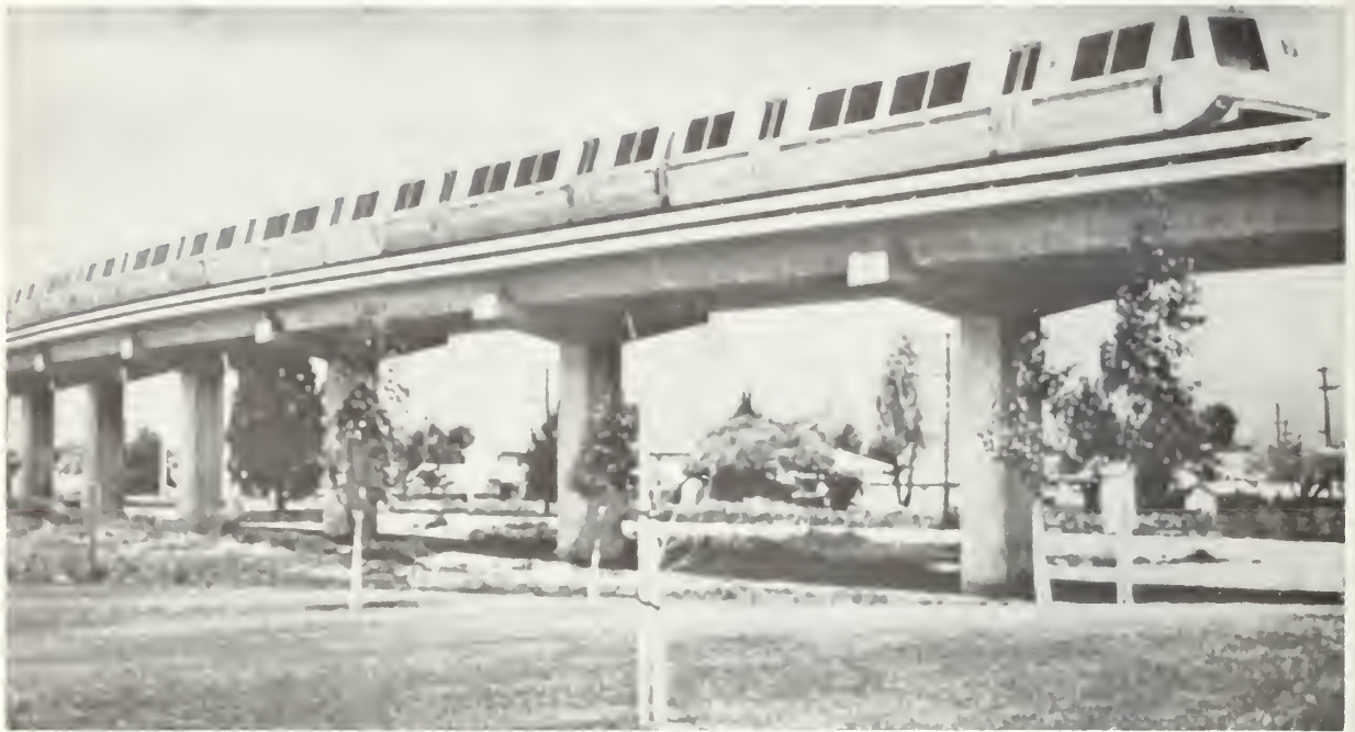
Figure 5-9. Typical BART Train (Six Cars Shown)
