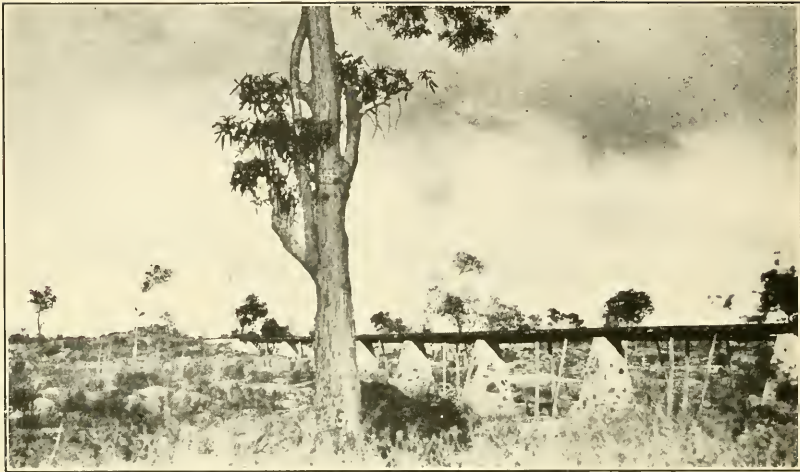
1. DRY CHANNEL CROSSED BY TROLLEY LEADING TO POWER PLANT
