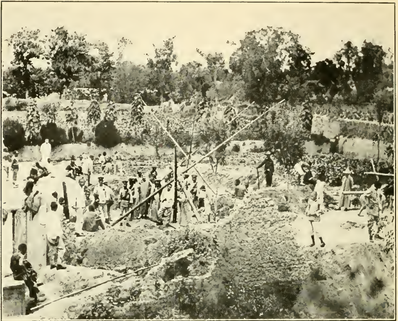
1. HSIEN-CH'ENG HSIEN. WORKMEN ABOUT MOUTH OF EXCAVATION SHAFT
