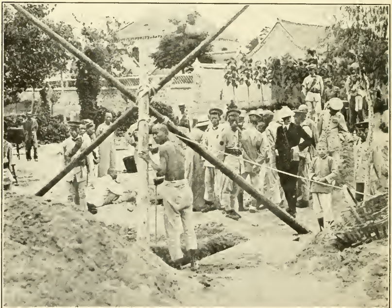
2. HSIEN-CH'ENG HSIEN. WORKMEN ABOUT MOUTH OF THE PIT, AND MR. WENLEY
