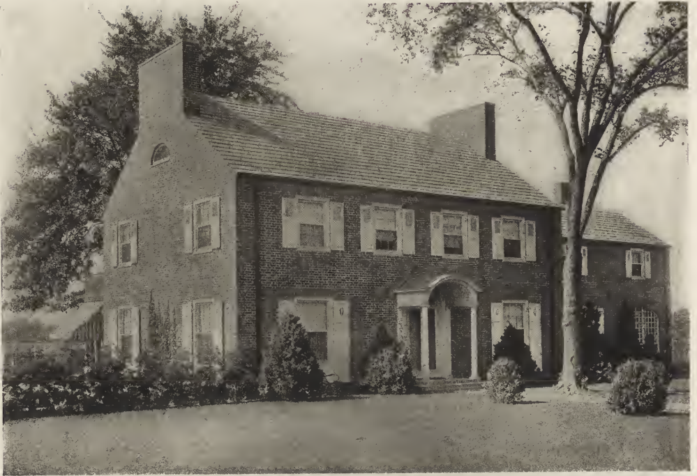
HOUSE OF MISS E. A. WATSON, WHITE PLAINS, N. Y. Delano & Aldrich, Architects.
