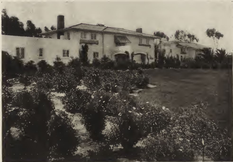
HOUSE OF J. W. SEFTON, JR., ESQ., WITH HOUSE OF MRS. HARRIETT SEFTON CAMPBELL IN DISTANCE, POINT LOMA, CAL. Will Sterling Hebbard, Architect.
