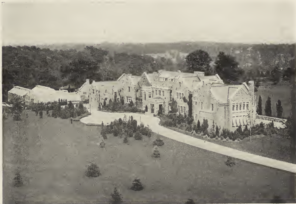
GENERAL VIEW—WEEK-END HOUSE OF ADOLPH LEWISOHN, ESQ., ARDSLEY, N. Y. Coulter & Westhoff, Architects.
