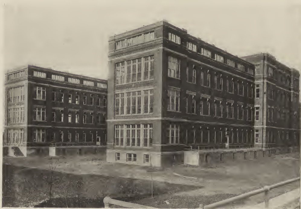
FIG. 12. REAR VIEW, WARD BUILDINGS "J" AND "K"—NEW GENERAL HOSPITAL, CINCINNATI, OHIO. Samuel Hannaford & Sons, Architects.
