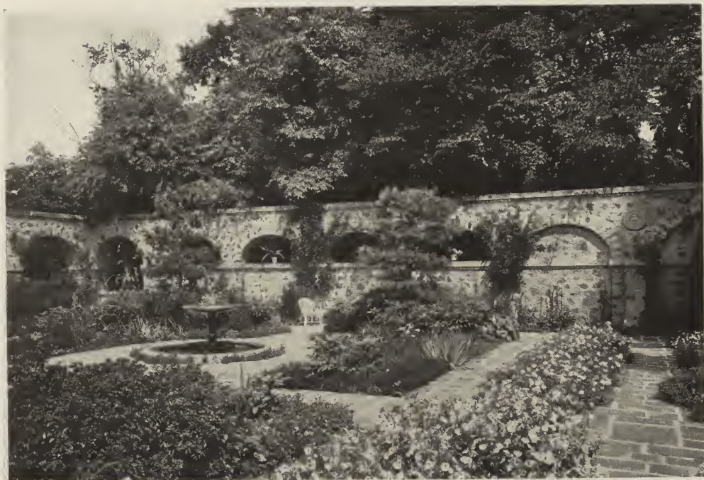
LOOKING ACROSS PATIO—RESIDENCE OF CHARLES S. WALTON, ESQ., ST. DAVIDS, PA. D. Knickerbacker Boyd, Architect.
