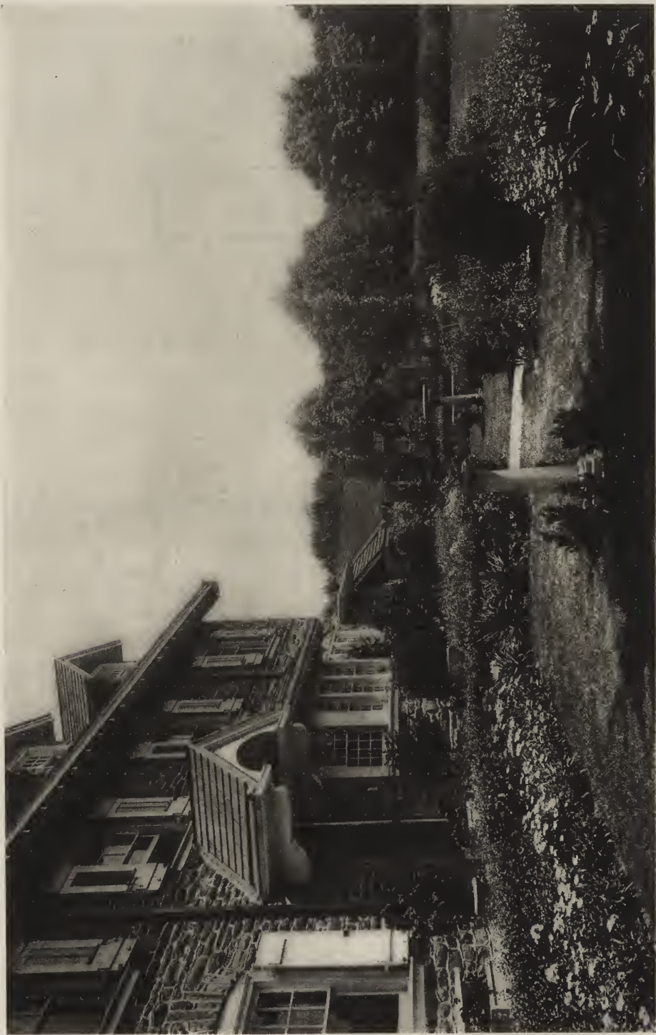
TERRACE—HOUSE OF RAEBURN CLARKE SMITH, ESQ., WYNNWOOD, PA. D. KNICKERBACKER BOYD, ARCHITECT.
