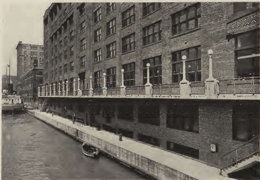
DETAIL—BUILDING OF REID, MURDOCH & CO., CHICAGO. George C. Nimmons, Architect.
