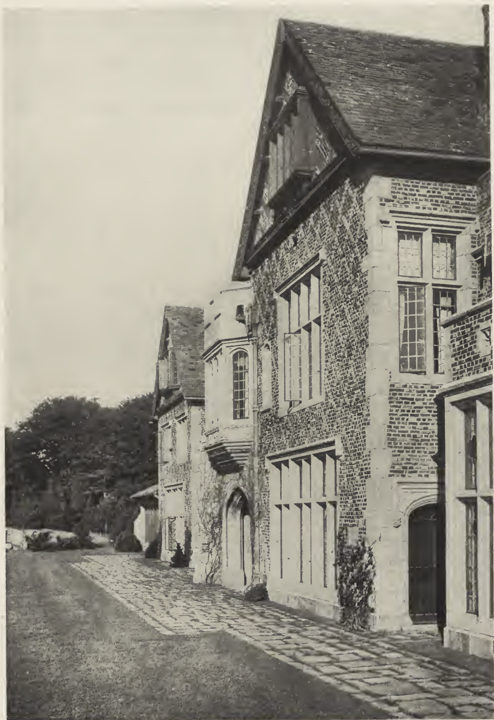
DETAIL OF SIDE TOWARD HARBOR—RESIDENCE OF STUART DUNCAN, ESQ., NEWPORT, R. I. JOHN RUSSELL POPE, ARCHITECT.
