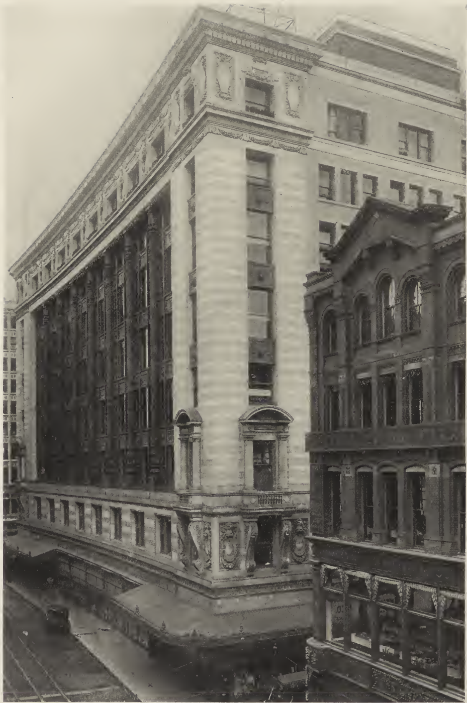
STORE OF WM. FILENE'S SONS CO., BOSTON, 1912, 1913. D. H. BURNHAM & CO. AND GRAHAM, BURNHAM & CO., ARCHITECTS.
