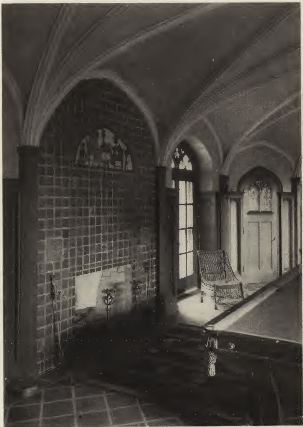
SIDE OF BILLIARD ROOM—RESIDENCE OF CHARLES S. WALTON, ESQ., ST. DAVIDS, PA. D. KNICKERBACKER BOYD, ARCHITECT.
