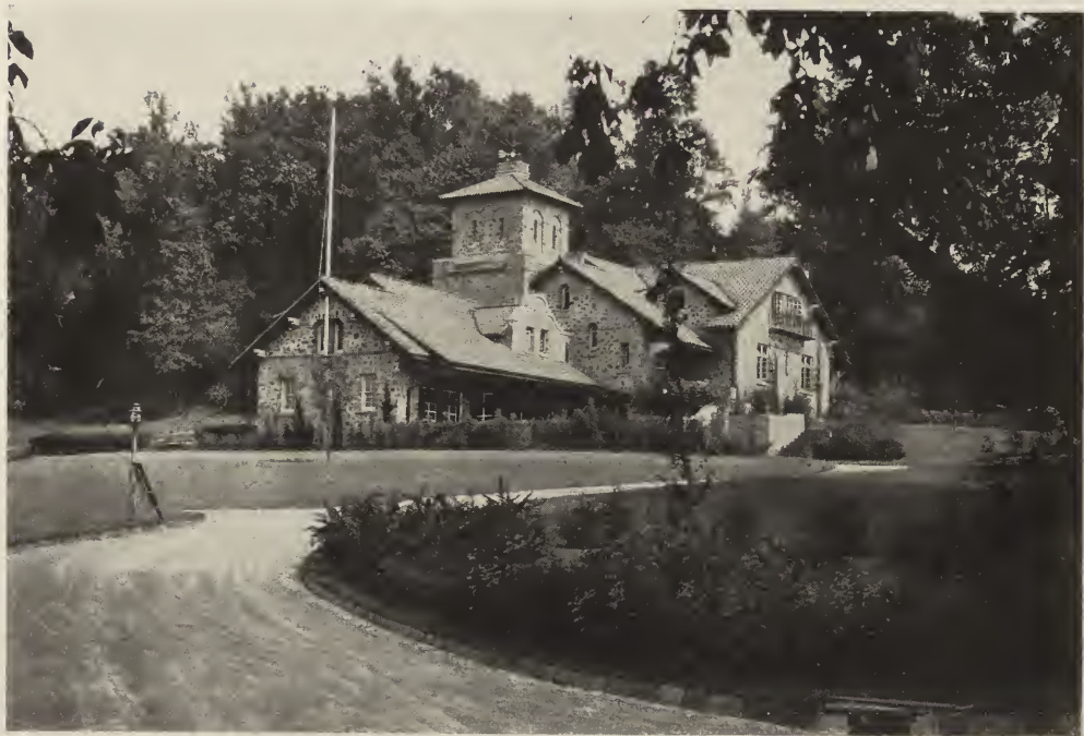
GARAGE—ESTATE OF CHARLES S. WALTON, ESQ., ST. DAVIDS, PA. D. Knickerbacker Boyd, Architect.
