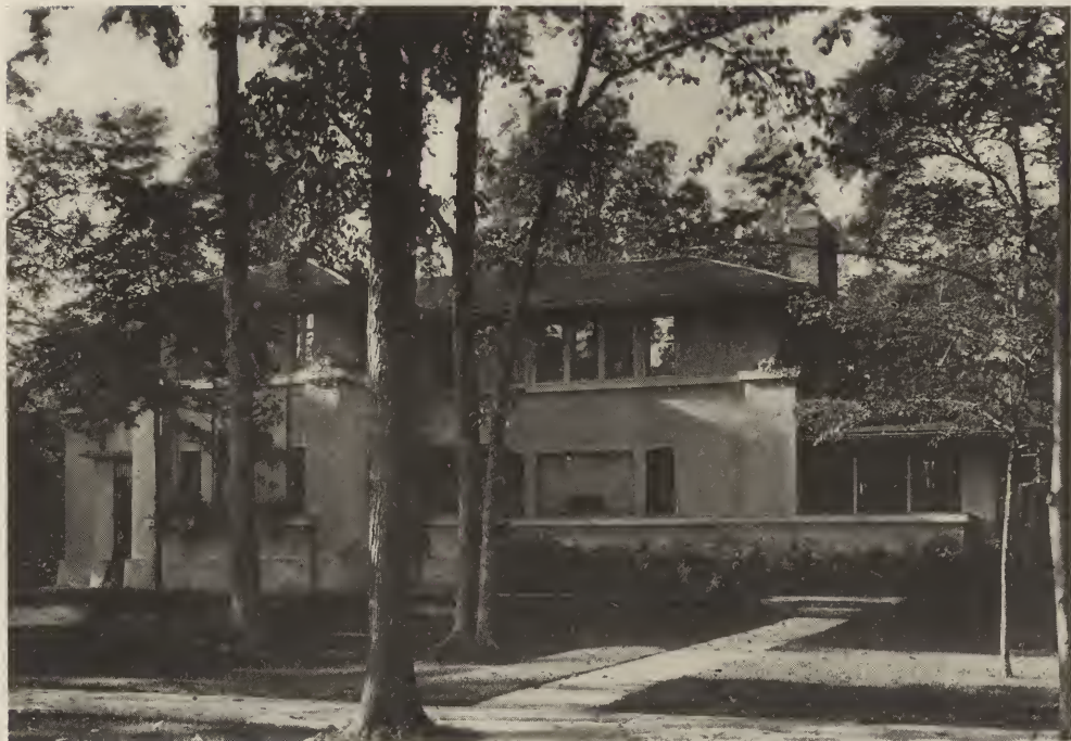
HOUSE OF JAMES A. GREEN, ESQ., KENILWORTH, ILL. Tallmadge & Watson, Architects.
