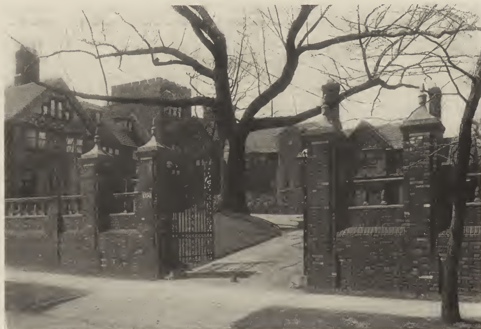
GATEWAY AND COURT—RESIDENCE OF F. E. DRURY, ESQ., CLEVELAND, OHIO. Frank B. Meade and James M. Hamilton, Architects.
