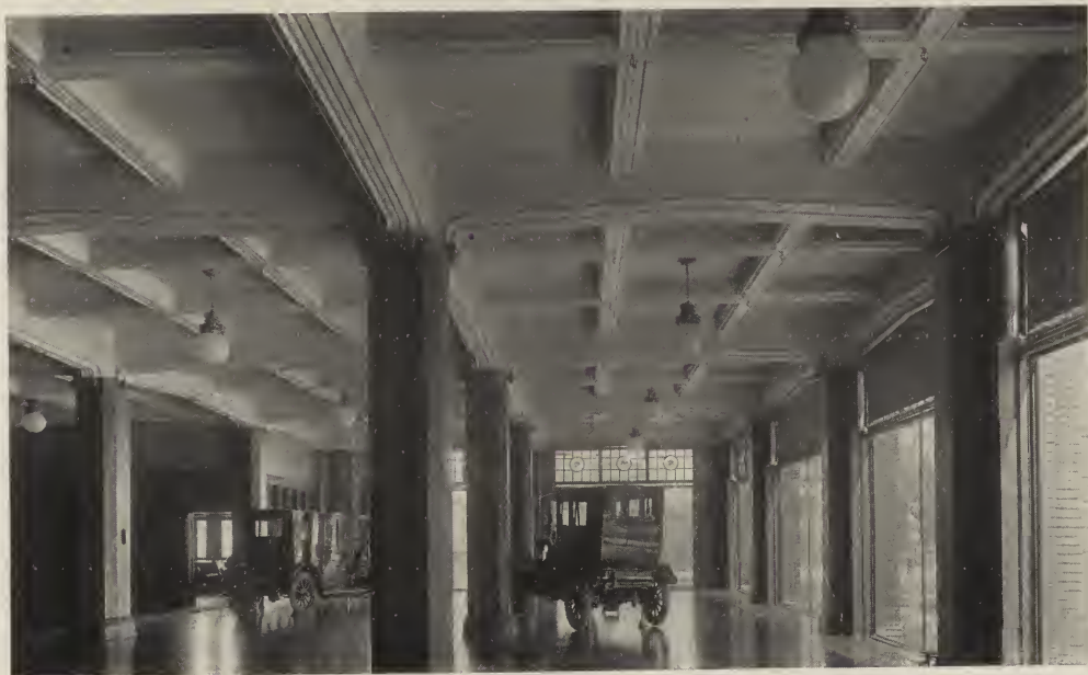
DISPLAY ROOM—BUILDING OF C. P. KIMBALL & CO., CHICAGO. George C. Nimmons, Architect.
