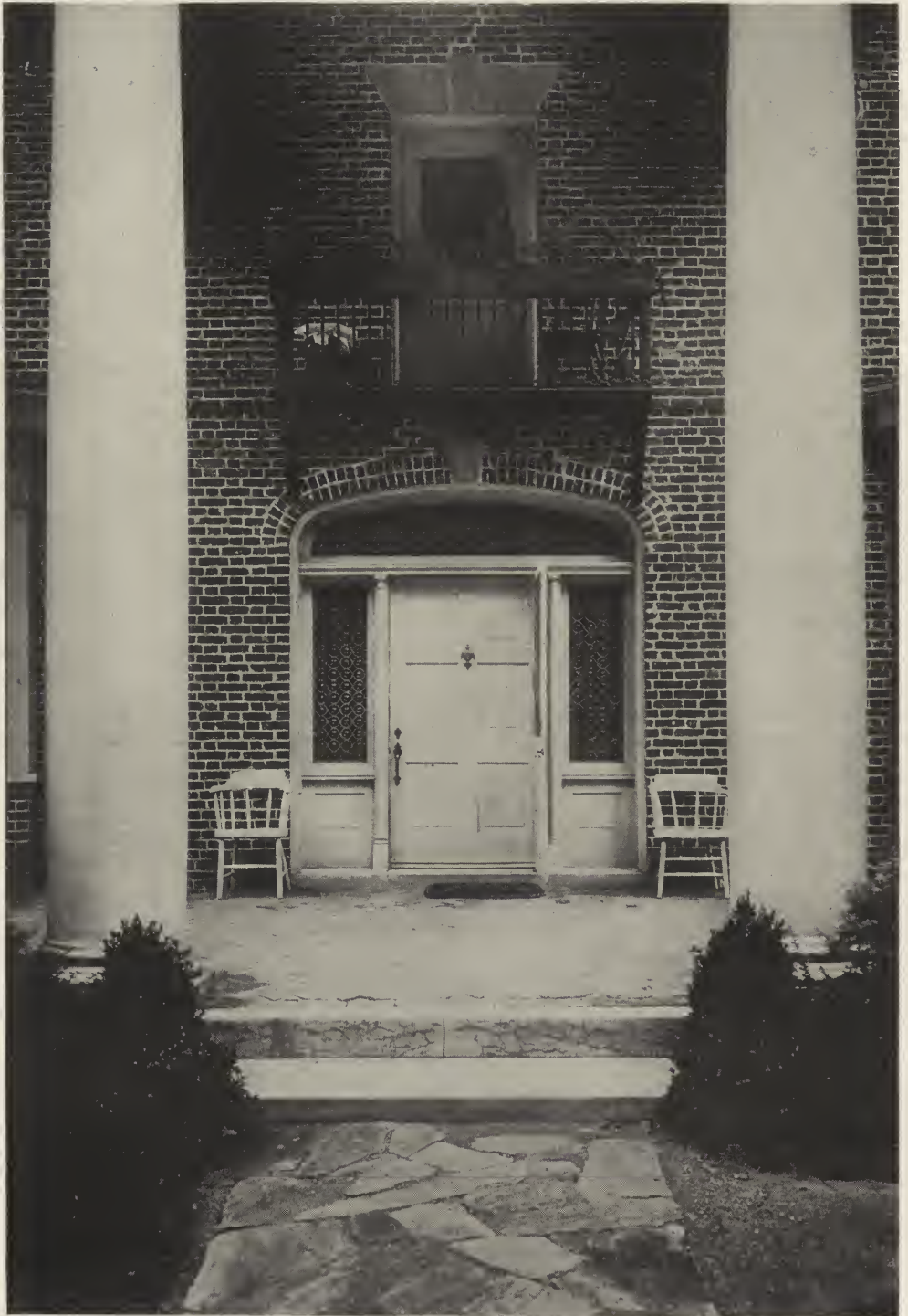
DOORWAY OF A HOUSE AT MT. AIRY, PA.
