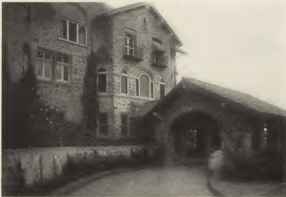
DINING ROOM BAY AND PORTE-COCHERE—RESIDENCE OF CHARLES S. WALTON, ESQ., ST. DAVIDS, PA. D. Knickerbacker Boyd, Architect.
