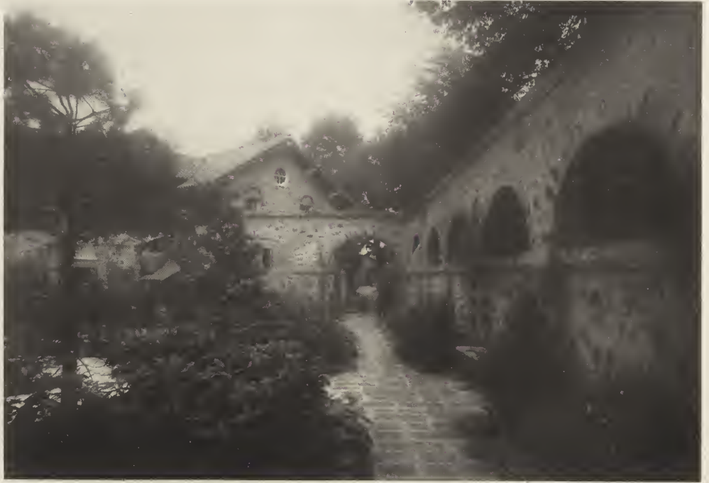
VIEW IN PATIO—RESIDENCE OF CHARLES S. WALTON, ESQ., ST. DAVIDS, PA. D. Knickerbacker Boyd, Architect.
