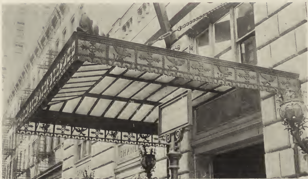
MARQUISE OF SHANLEY'S RESTAURANT, NEW YORK. Charles A. Platt, Architect.
