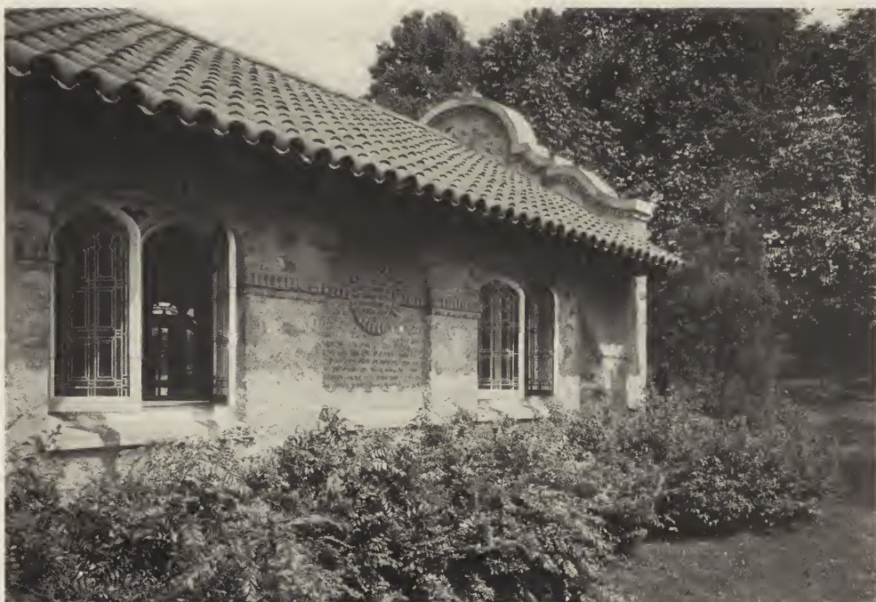
BILLIARD ROOM WING—RESIDENCE OF CHARLES S. WALTON, ESQ., ST. DAVIDS, PA. D. Knickerbacker Boyd, Architect.
