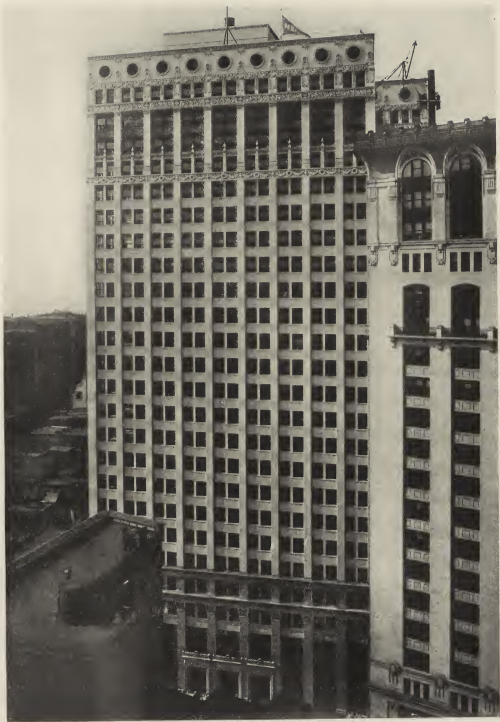
EIGHTY MAIDEN LANE, NEW YORK, 1911, 1912. D. H. BURNHAM & CO., ARCHITECTS.
