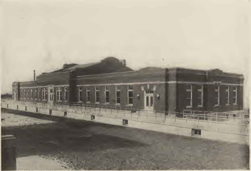
FIG. 9. KITCHEN BUILDING—NEW GENERAL HOSPITAL, CINCINNATI, OHIO. Samuel Hannaford & Sons, Architects.
