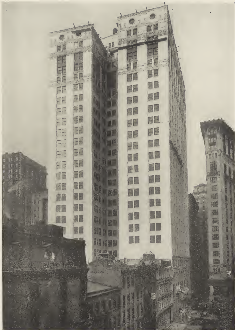
REAR VIEW—EIGHTY MAIDEN LANE, NEW YORK, 1911, 1912. D. H. BURNHAM & CO., ARCHITECTS.
