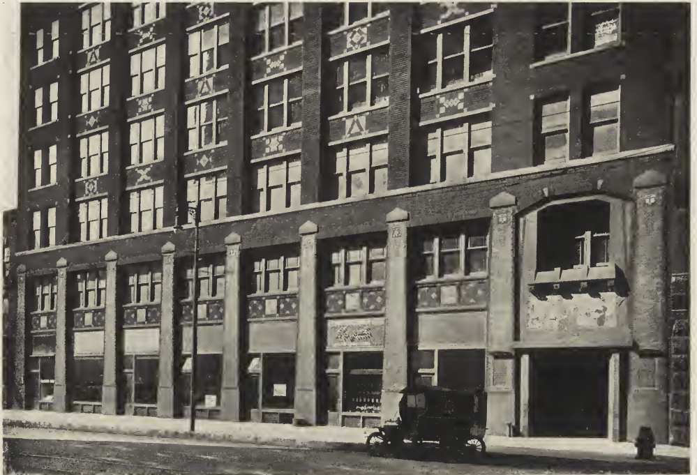
DETAIL—FRANKLIN BUILDING, CHICAGO. George C. Nimmons, Architect.
