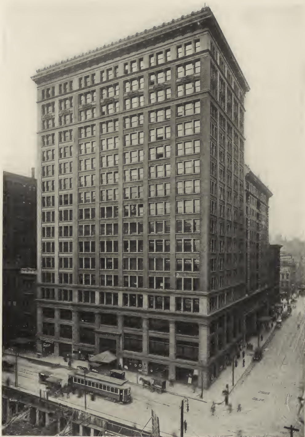
UNION SAVINGS BANK AND TRUST CO. BUILDING, CINCINNATI, OHIO, 1902, 1914. D. H. BURNHAM & CO. AND GRAHAM, BURNHAM & CO., ARCHITECTS.
