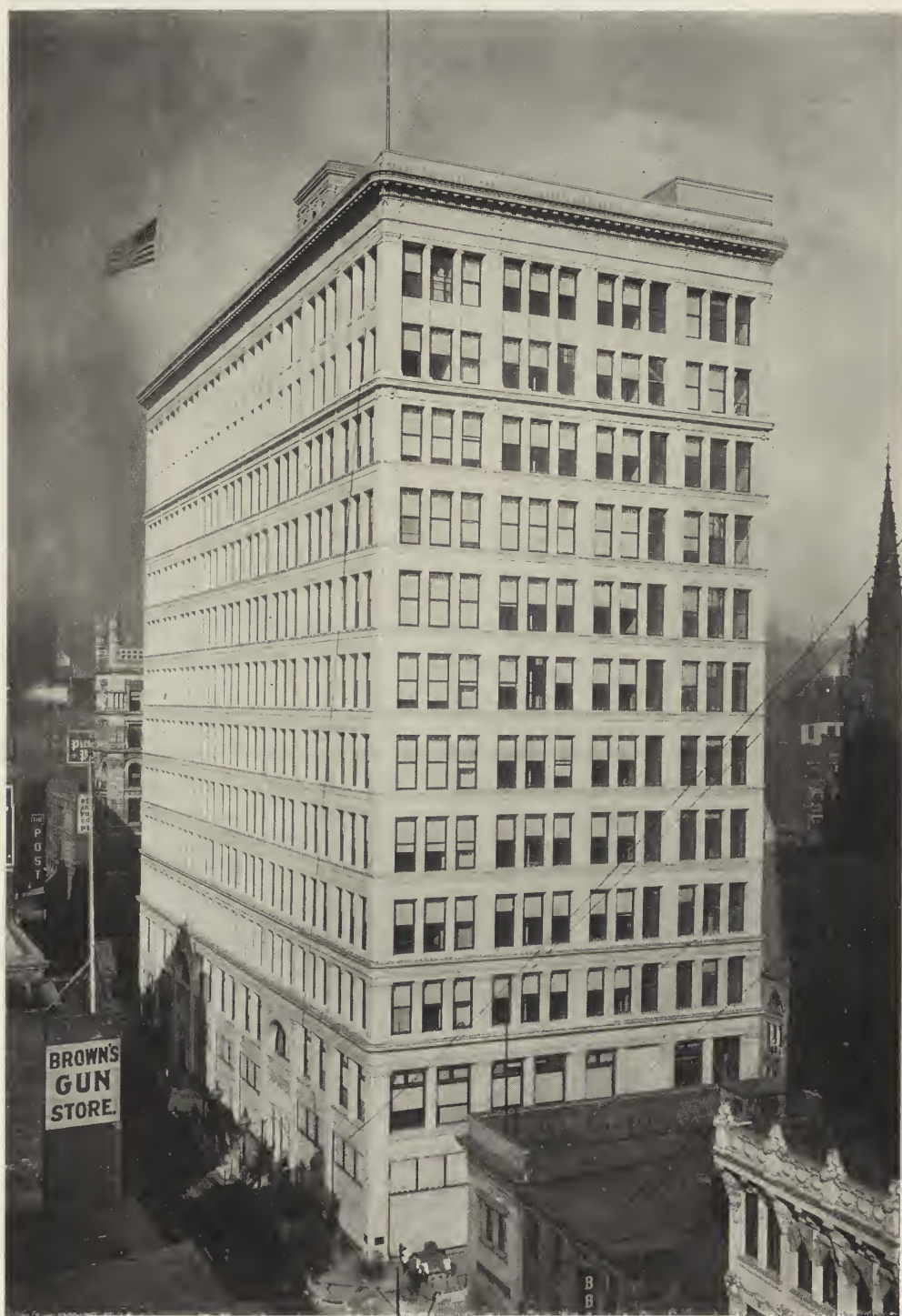
THE McCREERY STORE, PITTSBURGH, 1903. D. H. BURNHAM & CO., ARCHITECTS.
