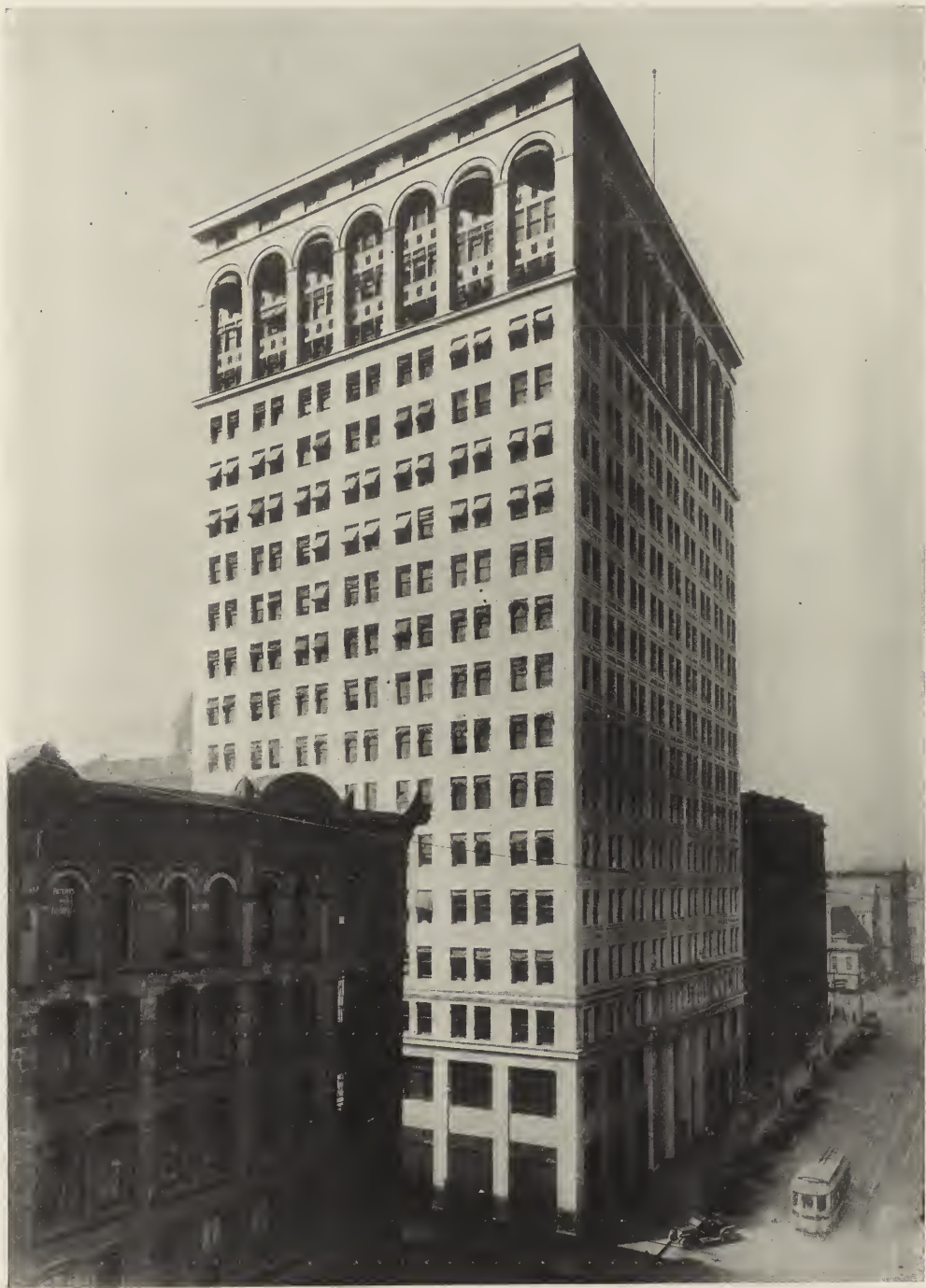
FORD BUILDING, DETROIT, MICH, 1908. D. H. BURNHAM & CO., ARCHITECTS.
