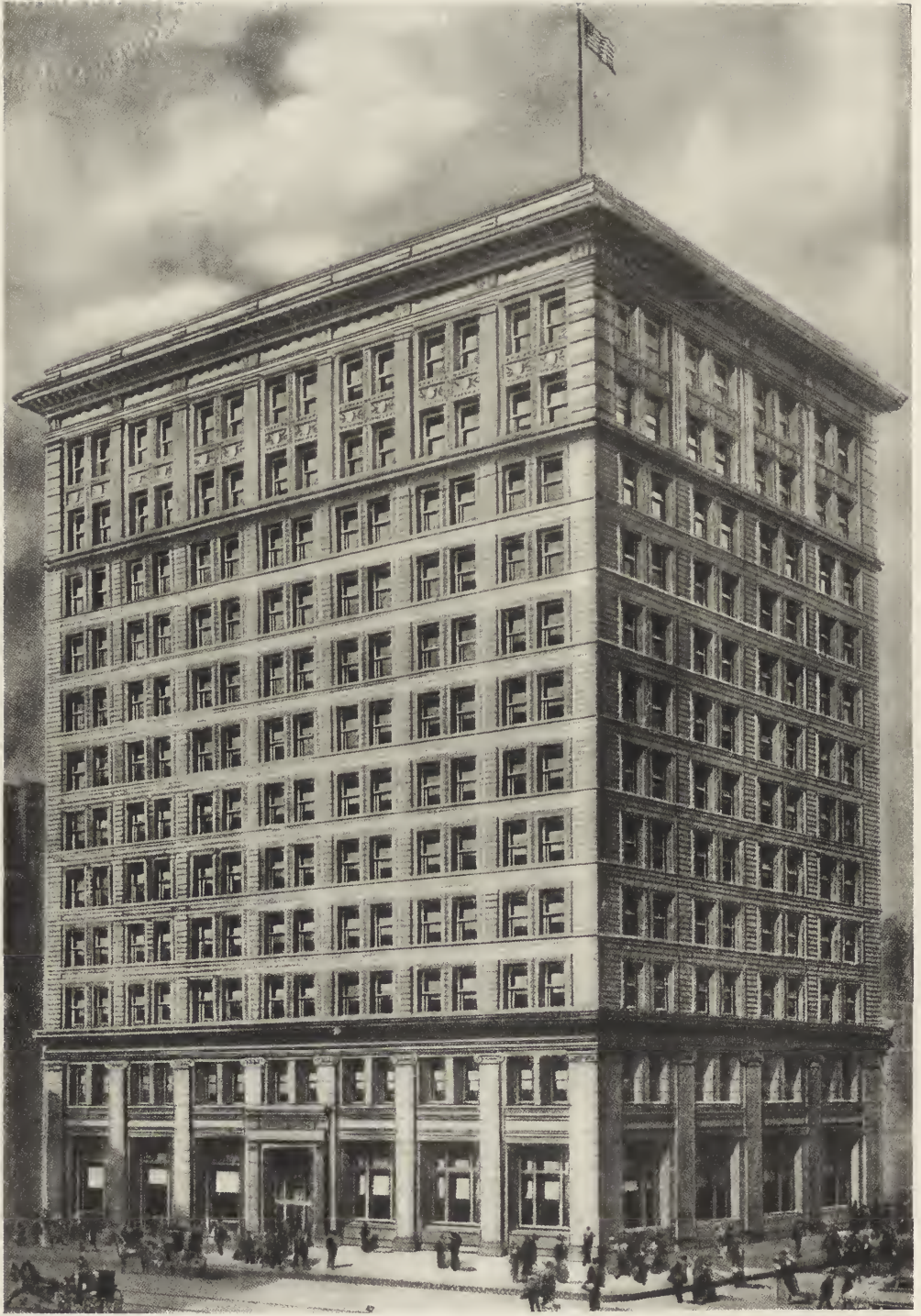
HIBERNIA BANK BUILDING, NEW ORLEANS, LA., 1903. D. H. BURNHAM & CO., ARCHITECTS.
