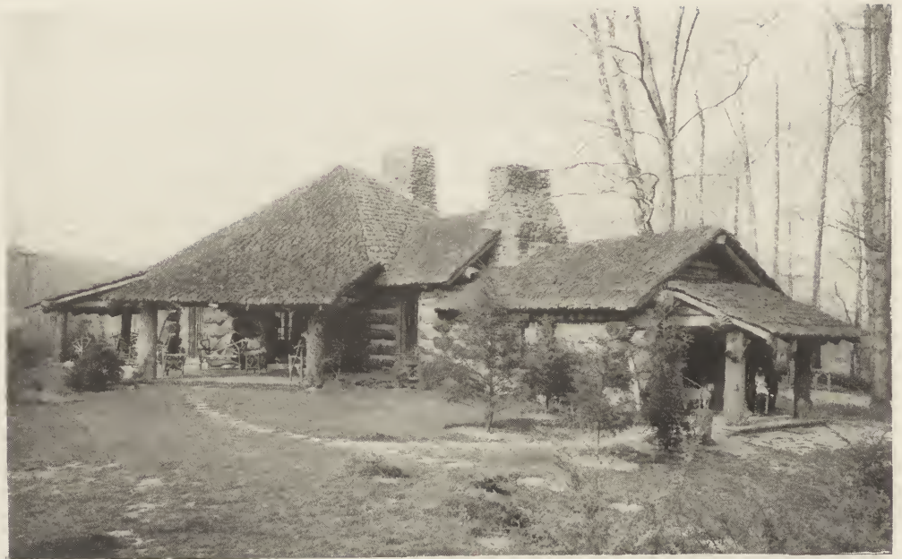
LOG CABIN—ESTATE OF CHARLES S. WALTON, ESQ., ST. DAVIDS, PA. D. Knickerbacker Boyd, Architect.
