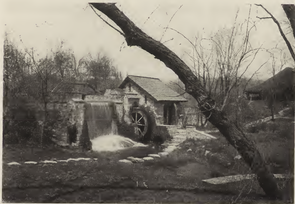
WATER WHEEL AND PUMP HOUSE—ESTATE OF CHARLES S. WALTON, ESQ., ST. DAVIDS, PA. D. Knickerbacker Boyd, Architect.
