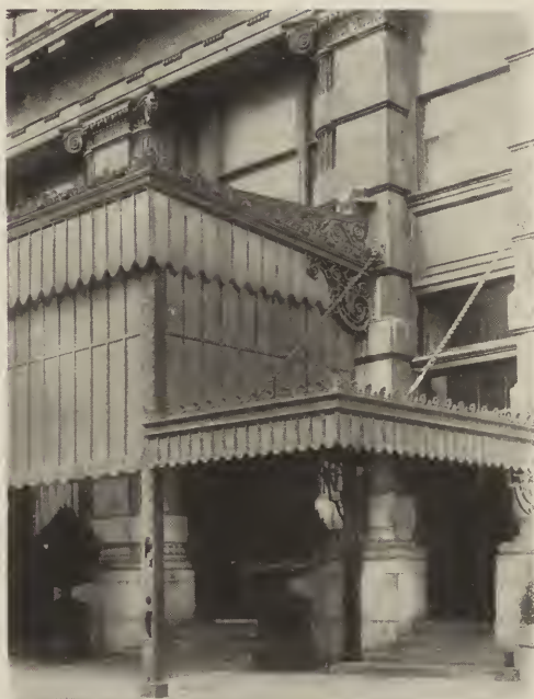
MARQUISE OF SHERRY'S, NEW YORK. McKim, Mead & White, Architects.
