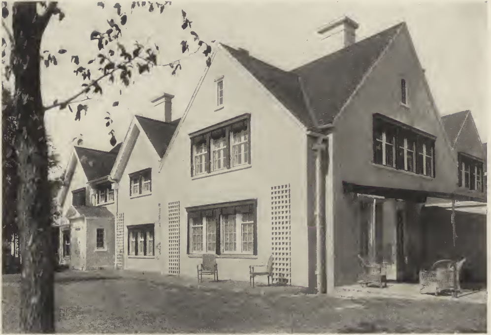
SOUTH TERRACE—HOUSE OF ARTHUR A. FOWLER, ESQ., PEAPACK, N. J. Hewitt & Bottomley, Architects.
