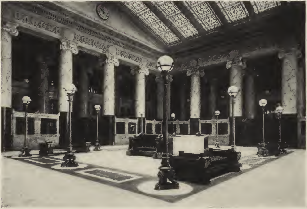
INTERIOR—PEOPLE'S GAS BUILDING, CHICAGO. D. H. Burnham & Co., Architects.
