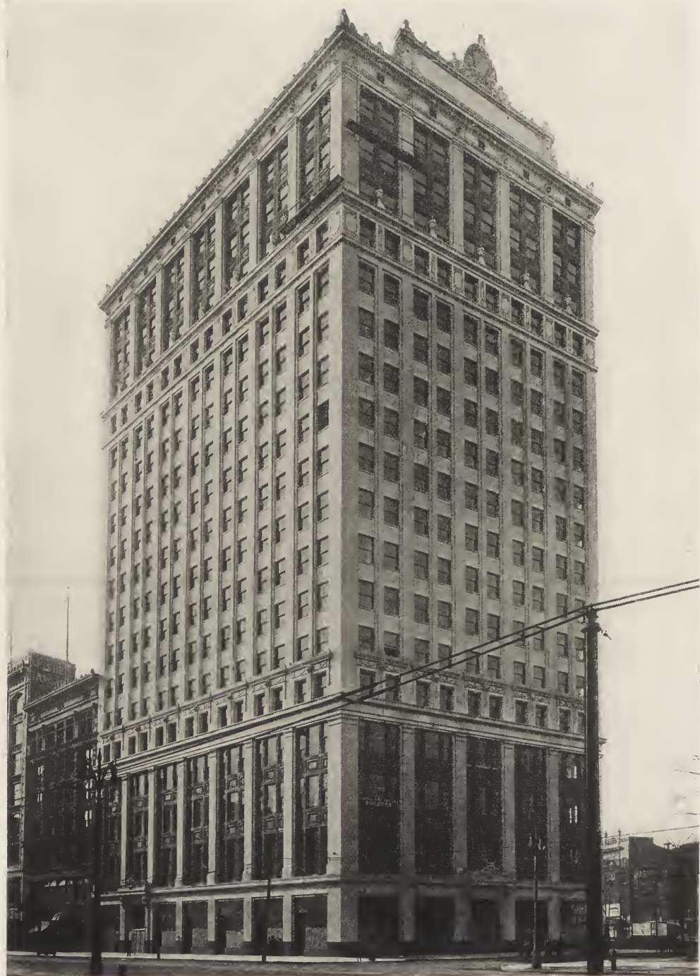
DAVID WHITNEY BUILDING, DETROIT, MICH. 1915. GRAHAM, BURNHAM & CO., ARCHITECTS.
