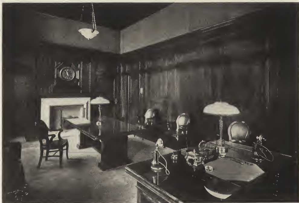
PRESIDENT'S ROOM—CONTINENTAL AND COMMERCIAL NATIONAL BANK, CHICAGO. D. H. Burnham & Co. and Graham, Burnham & Co., Architects.
