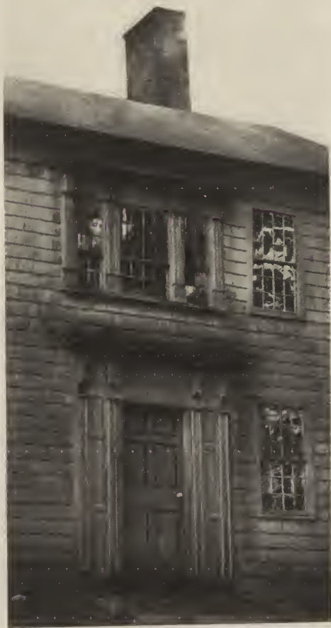
DOORWAY OF THE PLATT HOUSE, MERRYALL, CONN.
