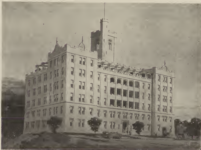
FIG. 22. GENERAL VIEW, OHIO VALLEY GENERAL HOSPITAL, WHEELING, WEST VIRGINIA. Edward F. Stevens, Architect.
