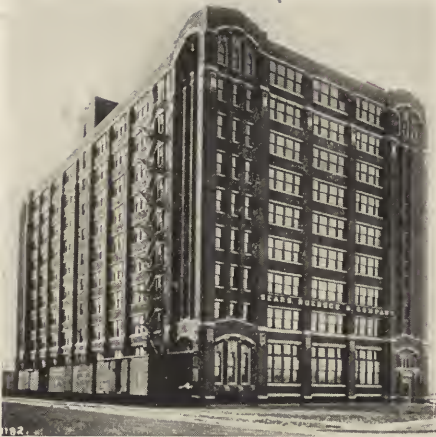
Completed First Unit.
