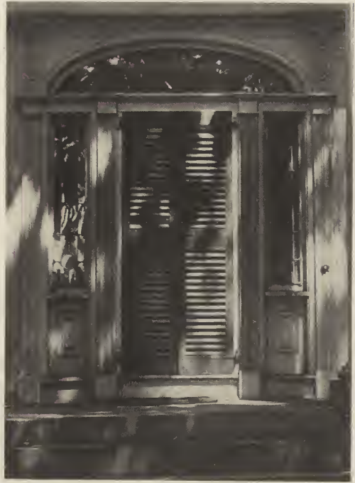
DOORWAY OF THE TAYLOR HOUSE, MILFORD, CONN.
