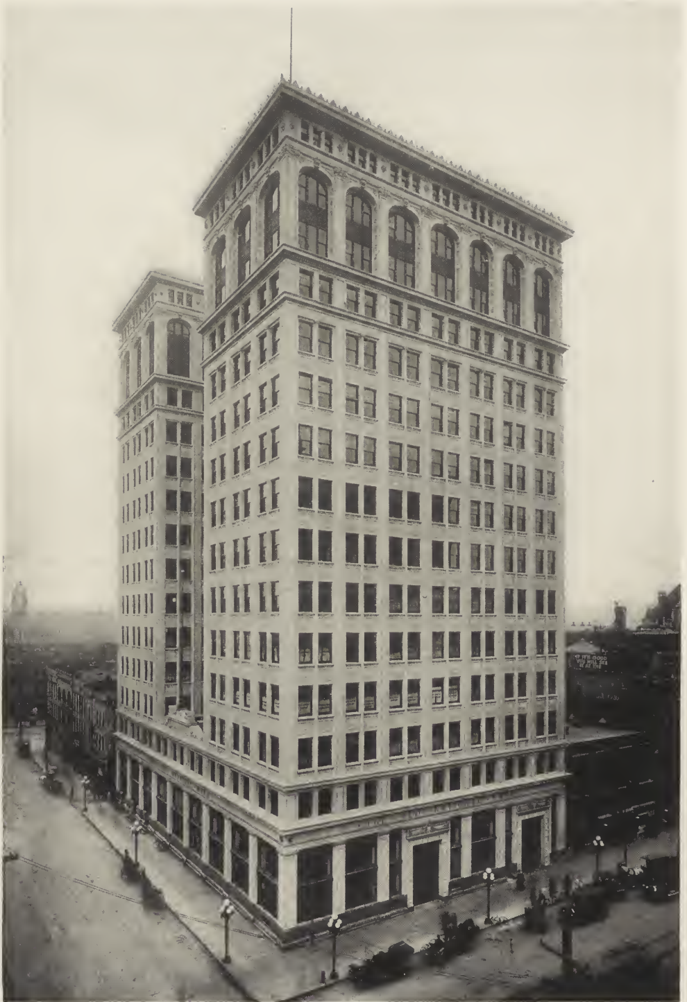
OLD NATIONAL BANK BUILDING, SPOKANE, WASH., 1910. D. H. BURNHAM & CO., ARCHITECTS.
