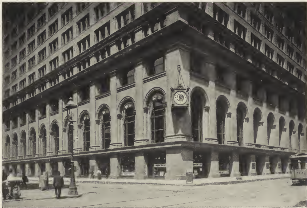
DETAIL—FIRST NATIONAL BANK, CHICAGO. D. H. Burnham & Co., Architects.
