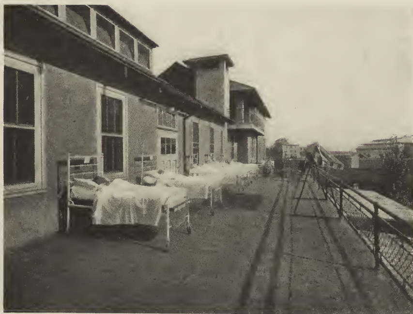
FIG. 21. AIRING BALCONY, PAVILION "C," PETER BENT BRIGHAM HOSPITAL, BOSTON, MASS. Codman & Despradelle, Architects.
