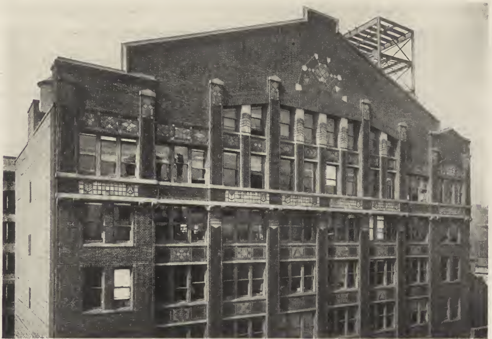
DETAIL—FRANKLIN BUILDING, CHICAGO. George C. Nimmons, Architect.
