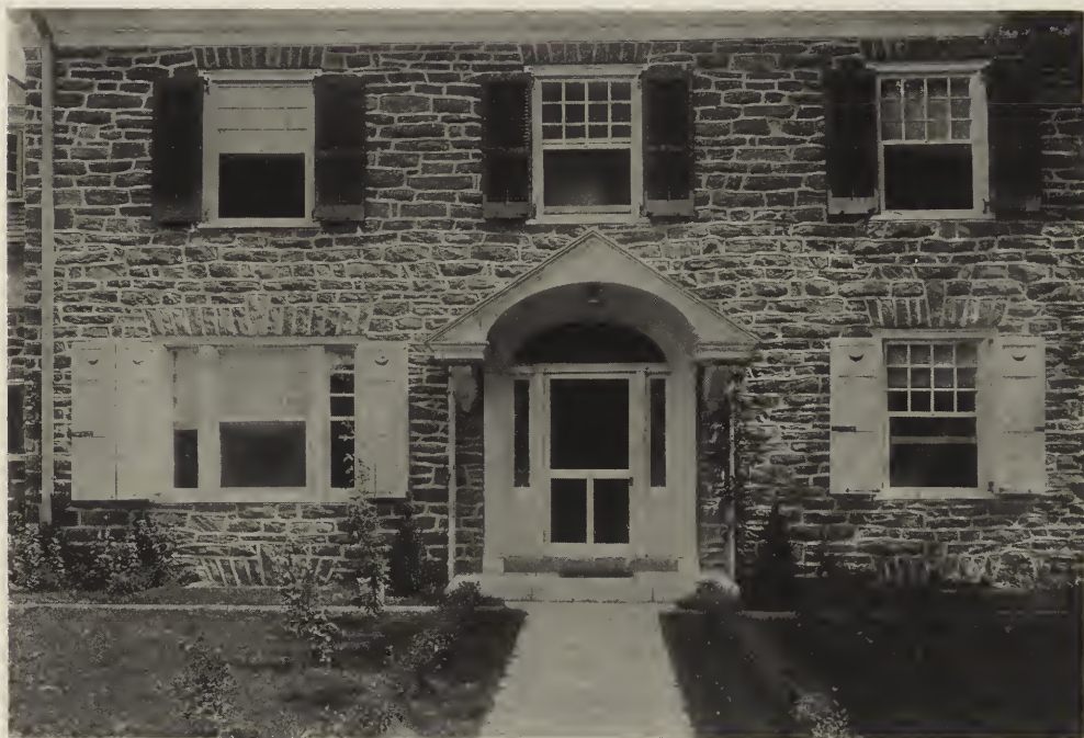
DOORWAY OF A HOUSE AT ARDMORE, PA. Horace Sellers, Architect.
