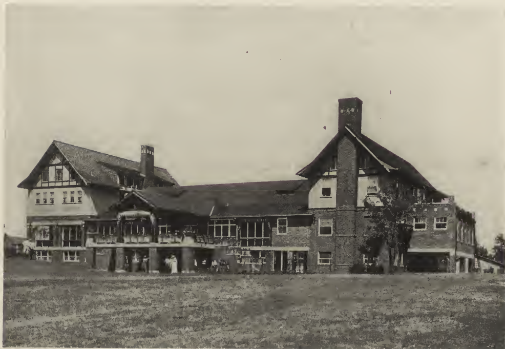
NORTH FRONT—EDGEWATER GOLF CLUB, CHICAGO. Hill & Woltersdorf, Architects.
