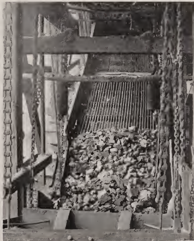
SCREENS AND BASKET AT NEW ENGLAND TIPPLE
