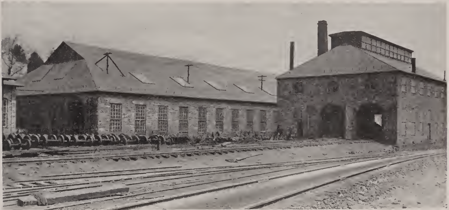
EXTERIOR OF "CUMBERLAND AND PENNSYLVANIA" SHOPS
