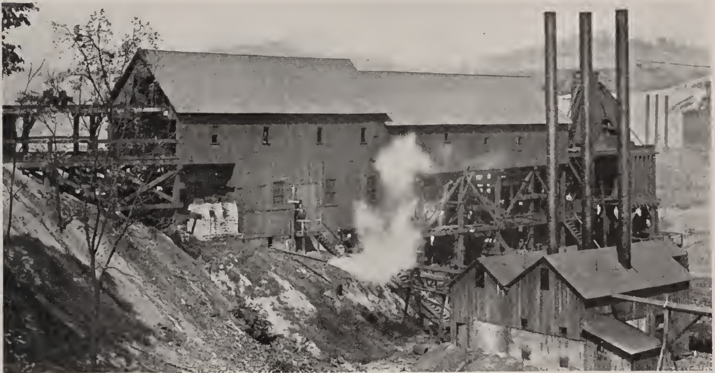
NEW ENGLAND TIPPLE AND POWER-HOUSE
