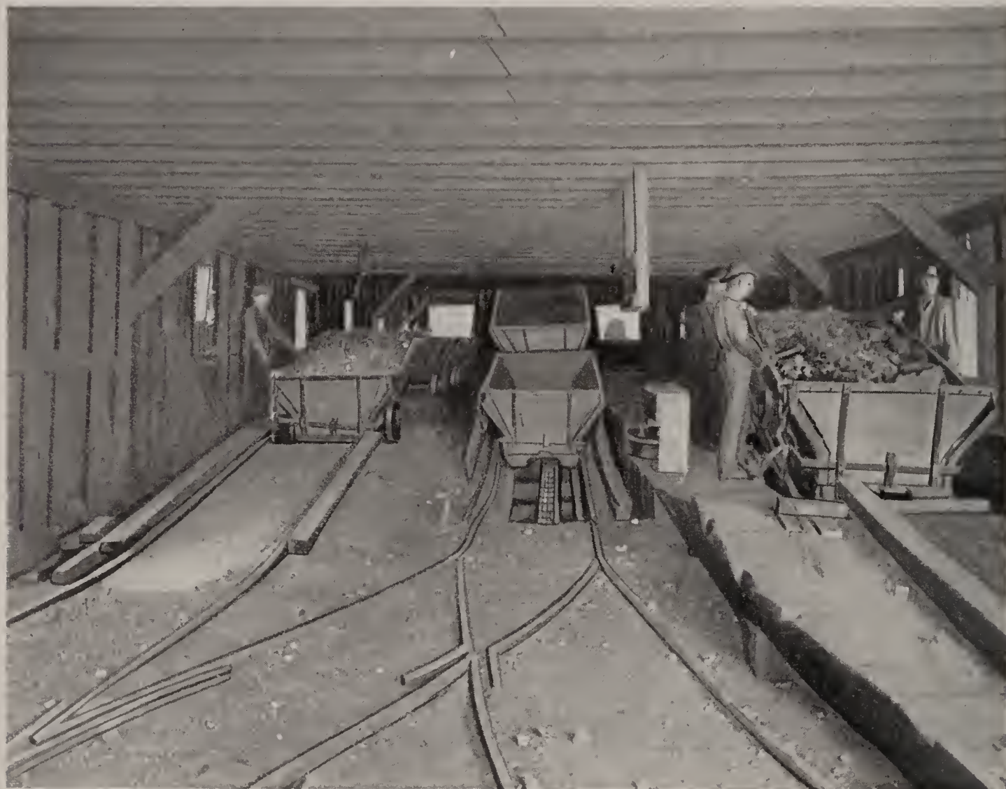
INTERIOR OF TIPPLE AT NEW ENGLAND MINE, SHOWING DUMPS AND CAR-HOISTS
