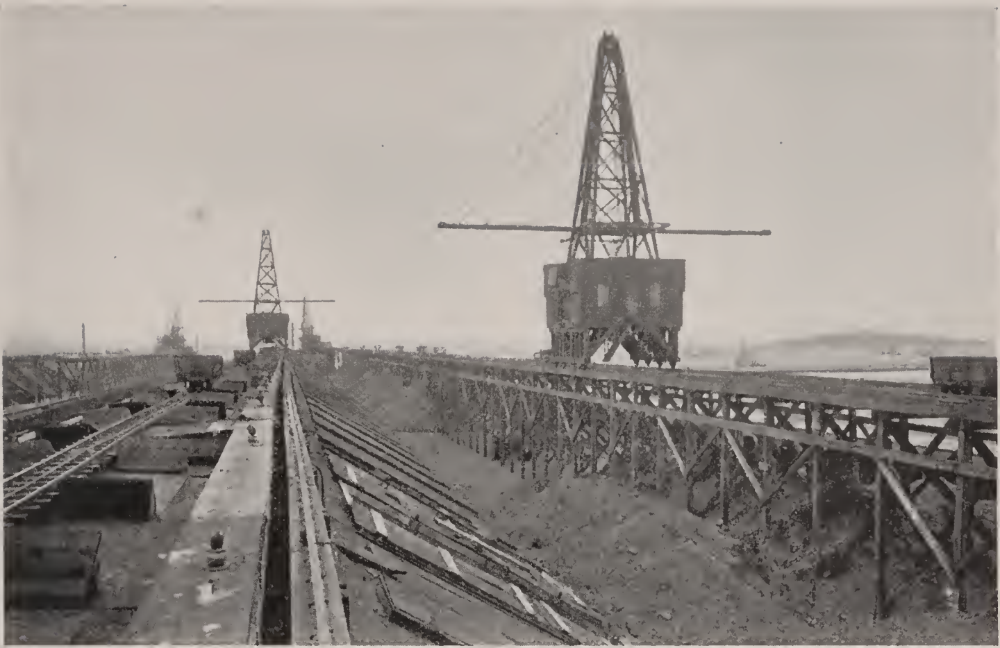
CANTILEVER TOWERS ON CONGRESS STREET WHARF, BOSTON
