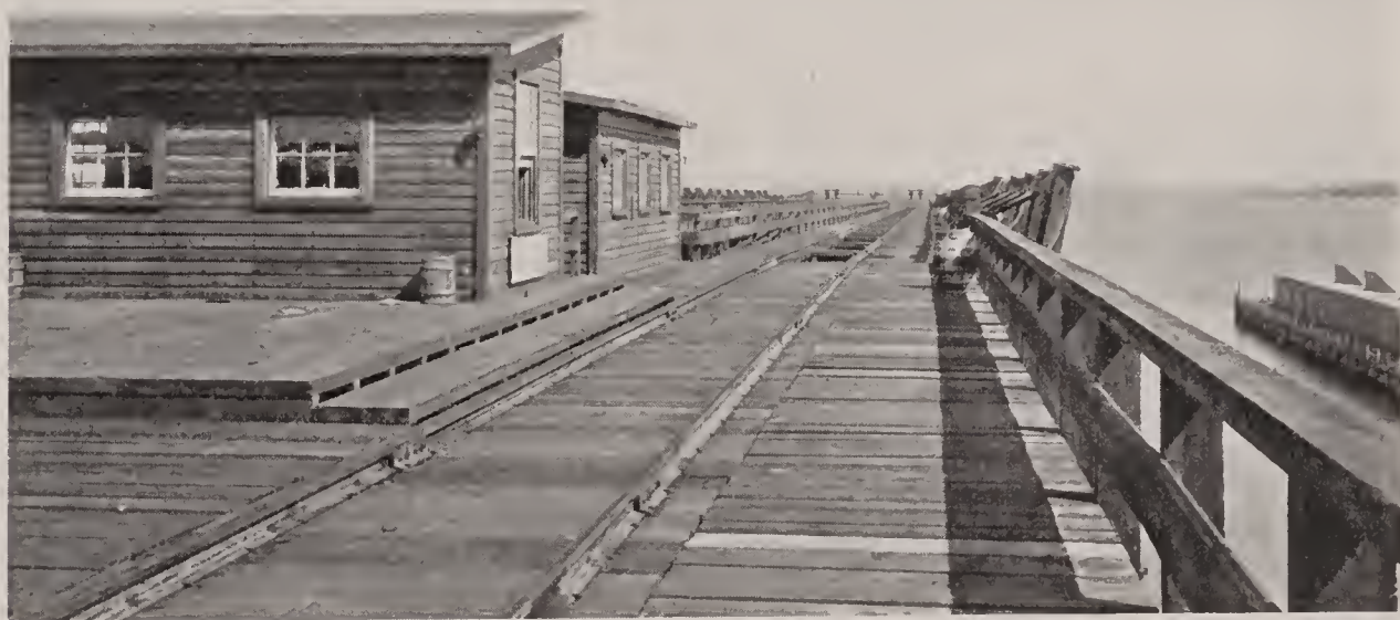
ONE OF THE 100-FOOT AUTOMATIC SCALES, CURTIS BAY COAL PIER, B. & O. R. R., BALTIMORE
