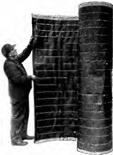
A large sheet of Linofelt which extends from one door of a refrigerator car around the end of car to the other door. Note the bound edges.
