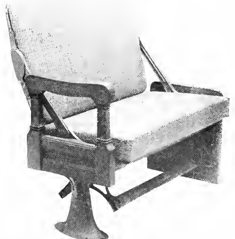
Fig. 1539—Universal Wakefield Reversing Seat with Turnover Reversing Action and Rattan Upholstery.
