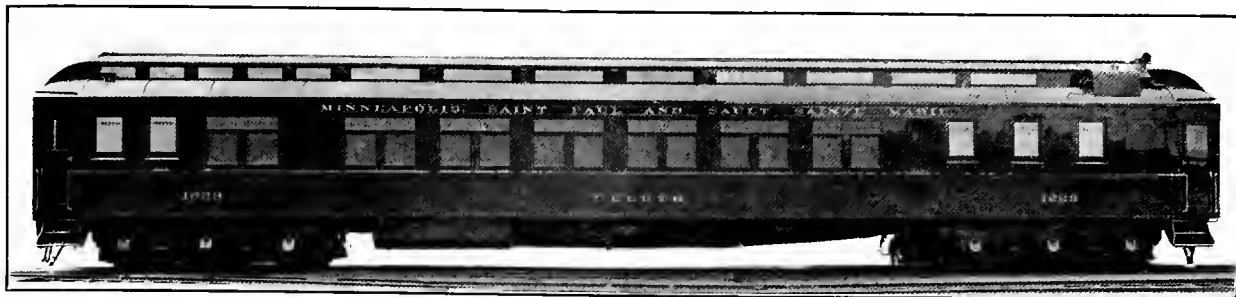
Fig. 180—Steel Vestibuled Sleeping Car. Weight, 142,300 lbs. Builder, The Barney & Smith Car Company.
