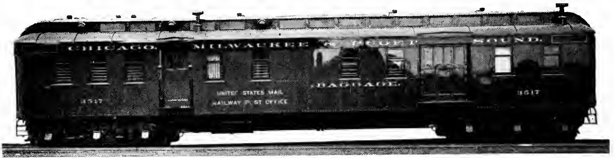
Fig. 134—Steel Baggage and Postal Car. Weight, 118,700 lbs.; Length Over Buffers, 63 ft. 2 \frac{7}{8} in. Builder, The Barney & Smith Car Co.
