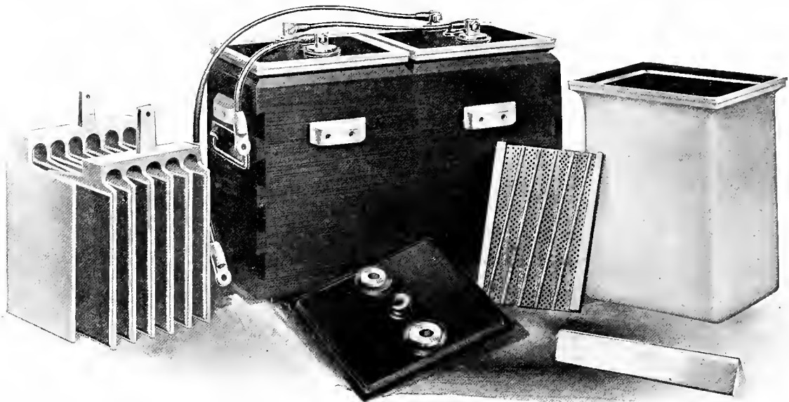
Fig. 2366—Willard Type P.T.L.-13 Train-Lighting Storage Battery and Parts, with Style A Connectors.
