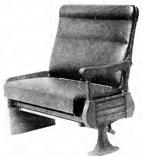
Fig. 1536—Wheeler Seat with Automatic Tilting Foot Rest and Leather Upholstery.
