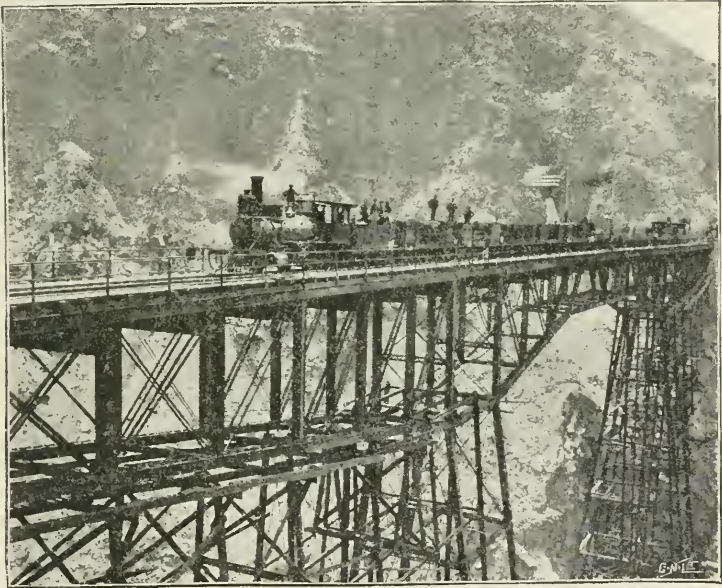
BRIDGE ON THE OROYA RAILWAY.
