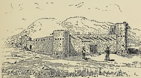
MEXICAN ADOBE HOUSE FORTIFIED AGAINST APACHE RAIDS.
