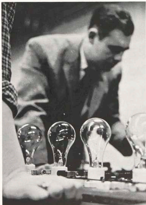
Determining how much current the load bank draws.
